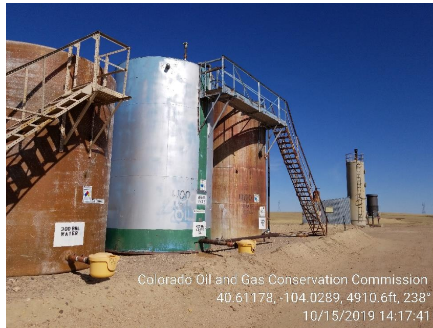
Photo 2 – Tank Battery – Crude Oil & Produced Water tanks are in poor paint condition. Refer to Rule 804
