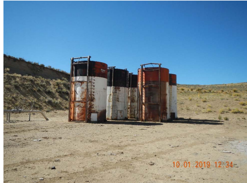
Photo 2. Frack tanks without containment and without labels.
