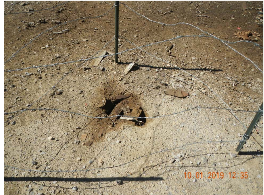
Photo 4. Open rathole and stained soil.
