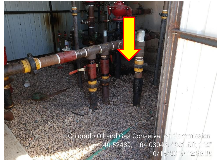
Photo 12 – Stained Soil at the Dump inside the Heater Shed
