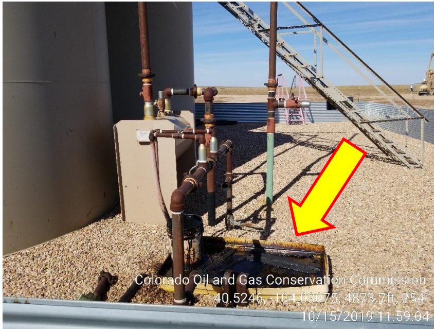
Photo 11 – Oily waste, trash inside containment, install Wildlife netting.
