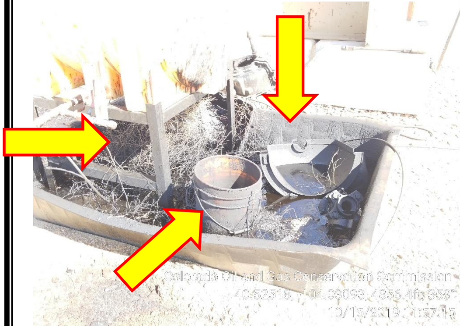
Photo 5 – Oily Waste, trash and debris inside containment.
