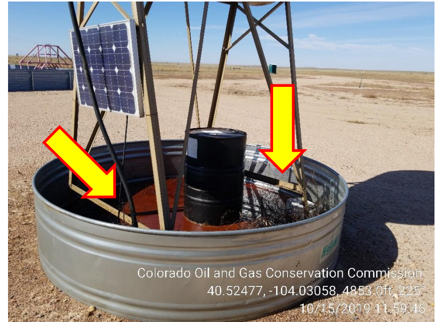
Photo 6 – Oily Waste and debris inside Containment. Install wildlife netting on Containment
