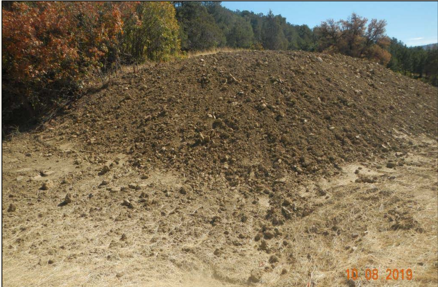
Photo 4. View of soil stockpile in the northeastern project area. Bare soil is not sufficiently protected/stabilized.
