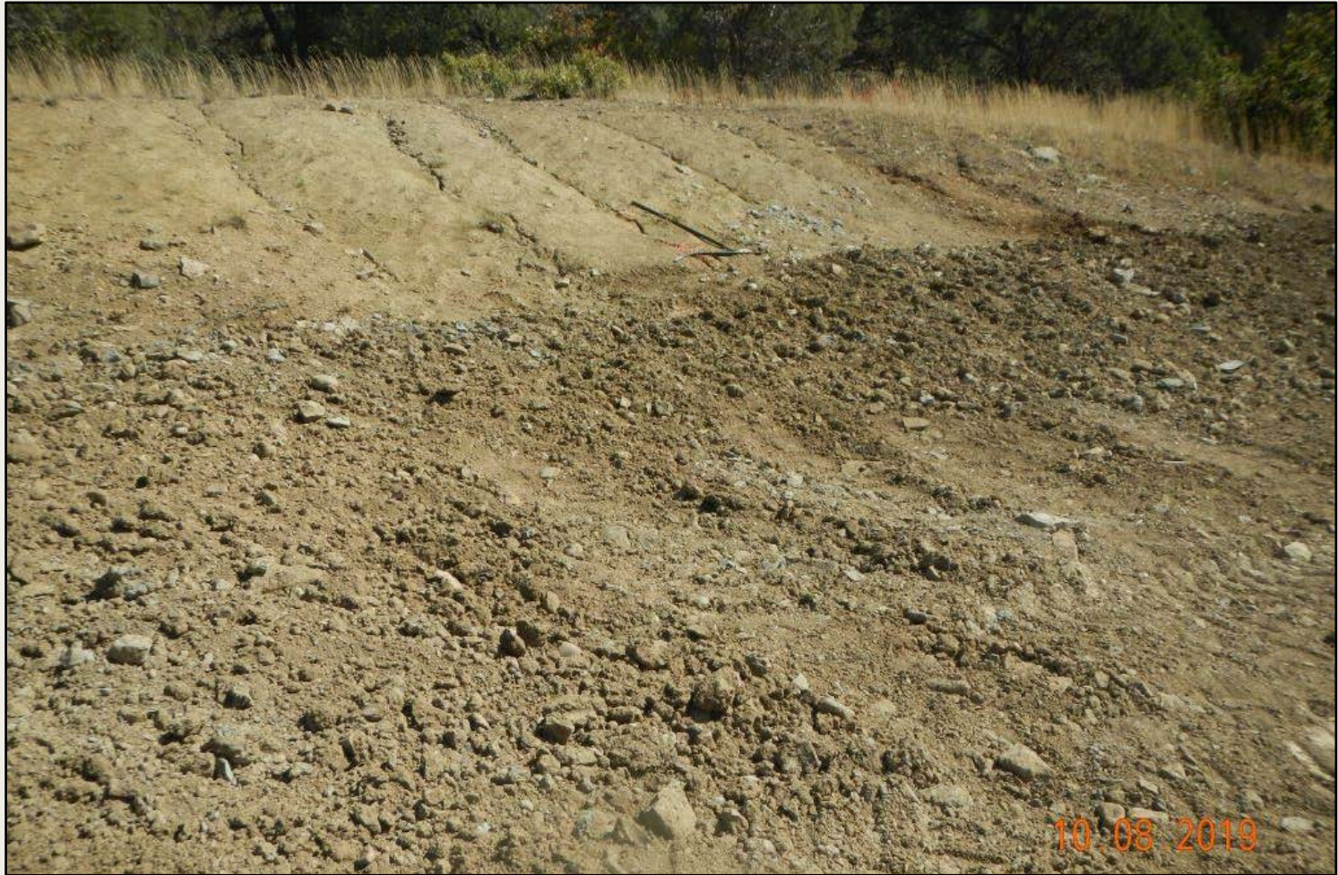
Photo 3. View of bare and eroding soils on the eastern cut-slope, not stabilized.
