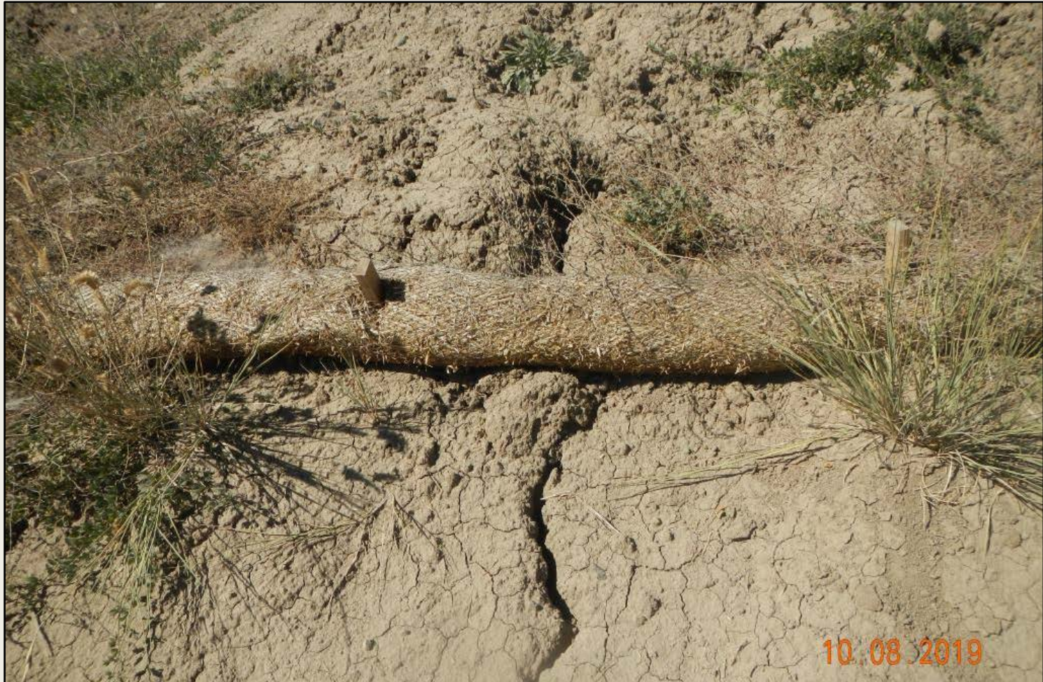
Photo 5. View of wattle at base of topsoil stockpile, that is not properly “trenched” into the soil, allowing runoff beneath the wattle and topsoil loss/sediment discharge.
