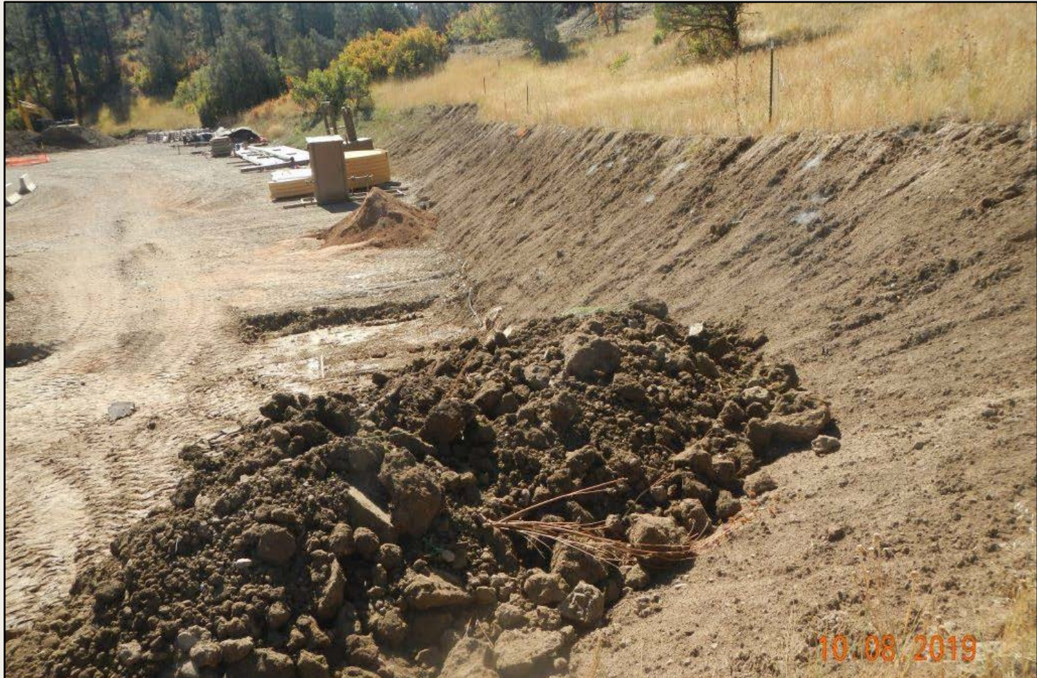
Photo 2. View of the western cut-slope from the northwestern corner facing southward. Slope appears too steep for vegetative stabilization.
