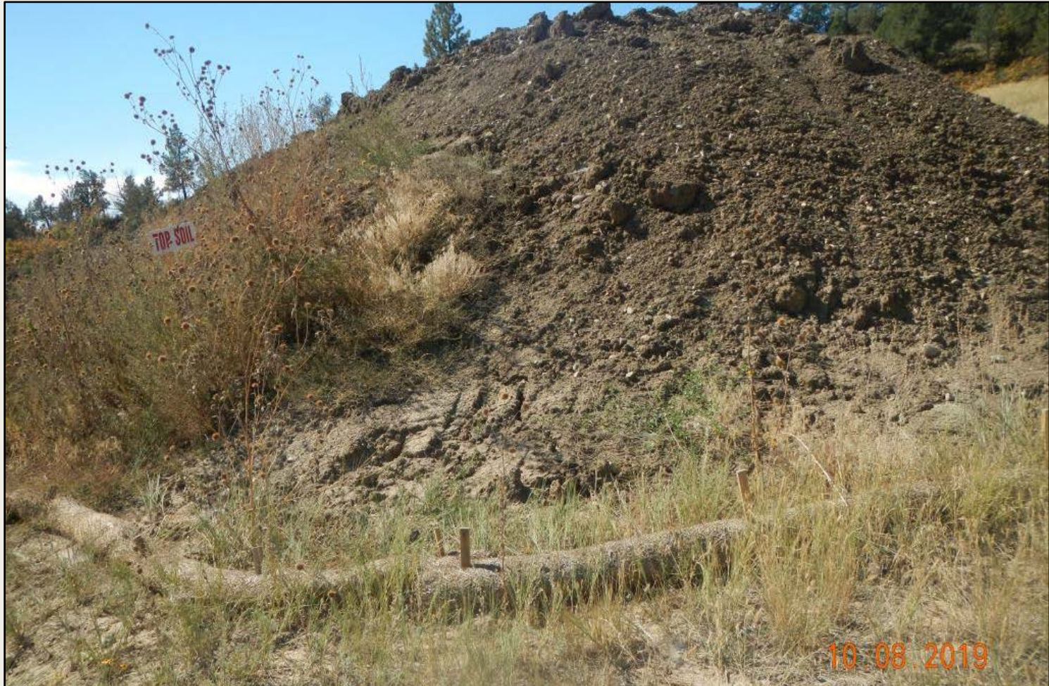
Photo 4. View of topsoil stockpile in the northern project area. Topsoil is not sufficiently protected, as tall pile is too deep to retain microbial activity, soil is bare or supporting weeds and exposed to erosion, and wattle surrounding the pile is not sufficient to prevent runoff of topsoil.
