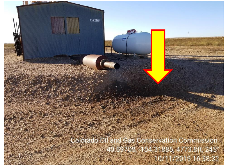
Photo 4 – Stained Soil at Engine Exhaust
