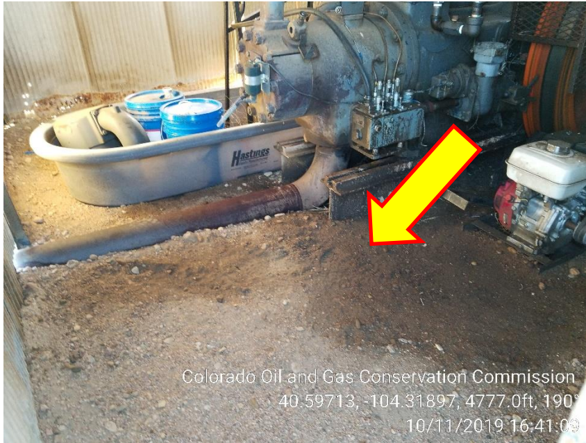
Photo 5 – Stained Soil at Engine
