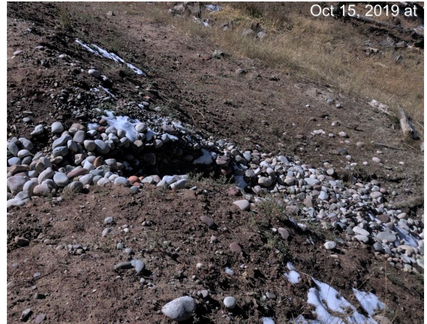
Washed out gravel on location drainage.
