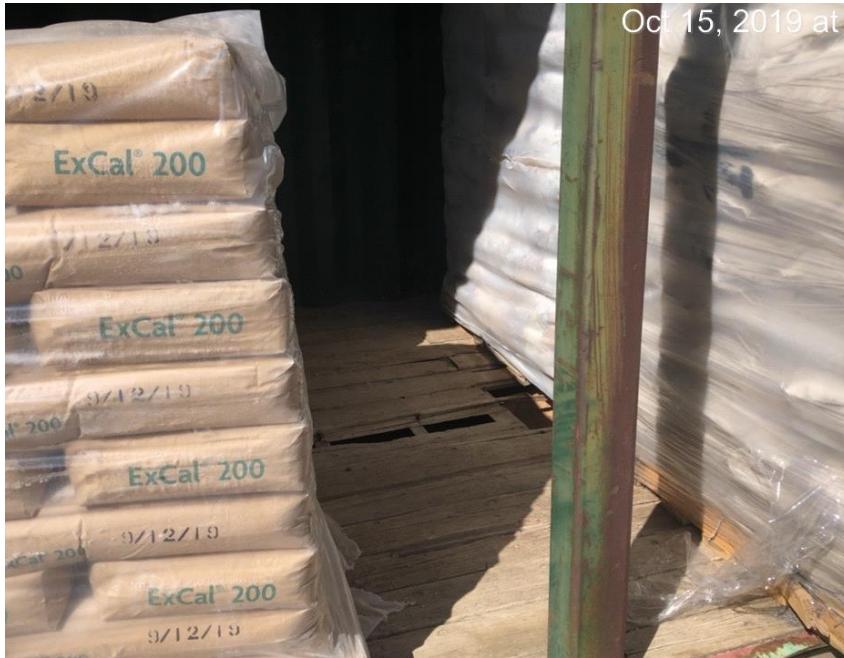
Spill materials in chemical storage box with damaged floor.
