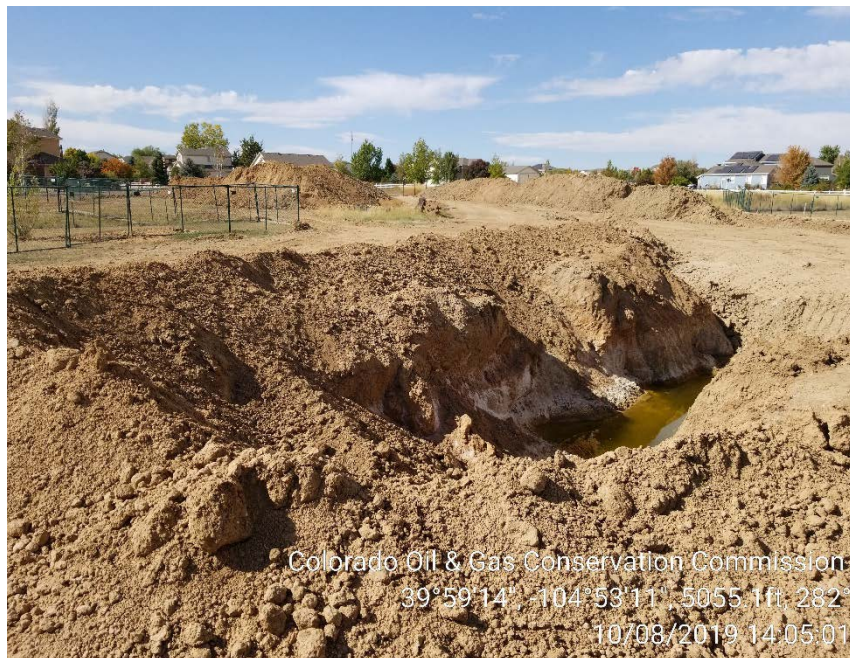
Photo 5: Ground water has infiltrated open excavation.
