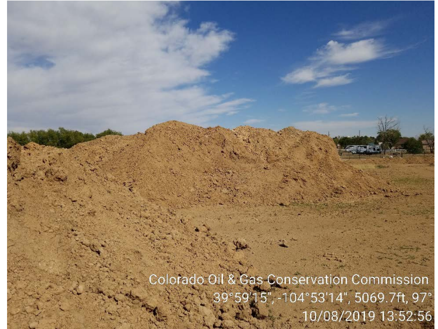
Photo 4: Spoil Pile without storm water BMPs.
