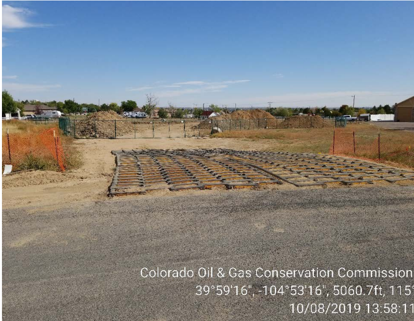
Photo 1: Track-out control mat and perimeter fence gate.
