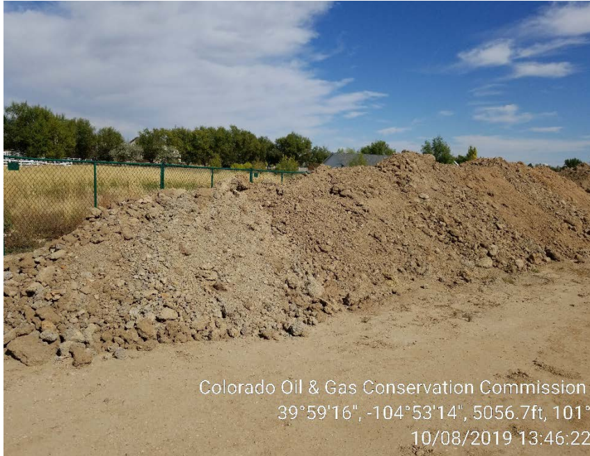
Photo 3: Spoil pile without storm water BMPs.
