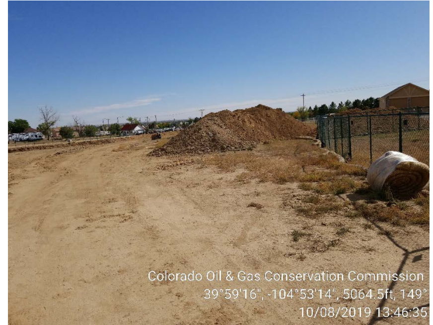
Photo 2: Spoil pile. Wattles have been deployed at some places inside the perimeter fence, but do not cover the entire perimeter.
