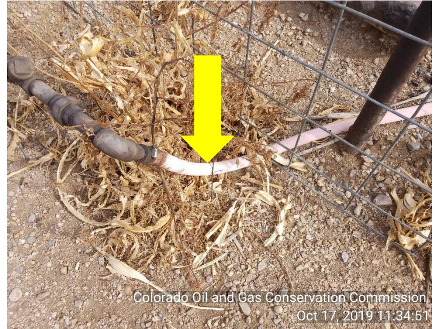
Photo 4 red fuel gas line weather beaten and leaking
