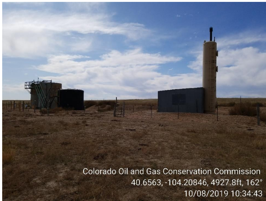
Photo 1 – Tank Battery
