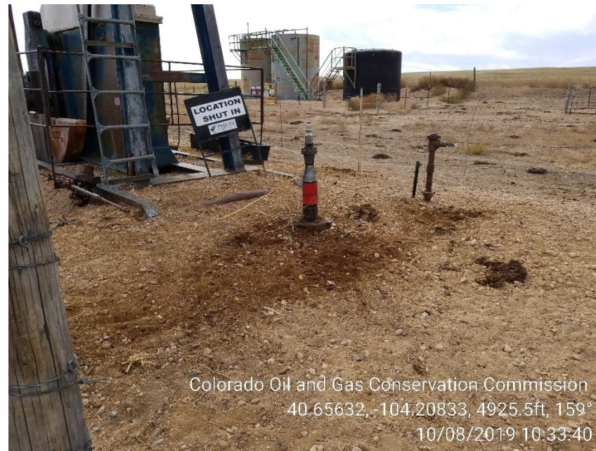
Photo 2 – Stained Soil at Wellhead
