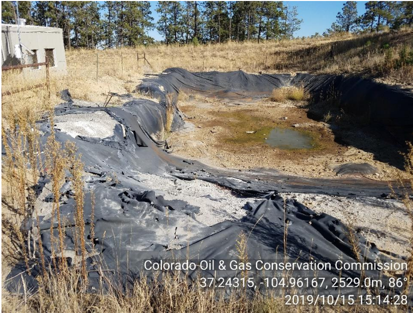
PHOTO 3: PIT LINER COMPROMISED. MAINTAIN PIT LINER AS PER RULE 904. CA DATE 11-15-19
