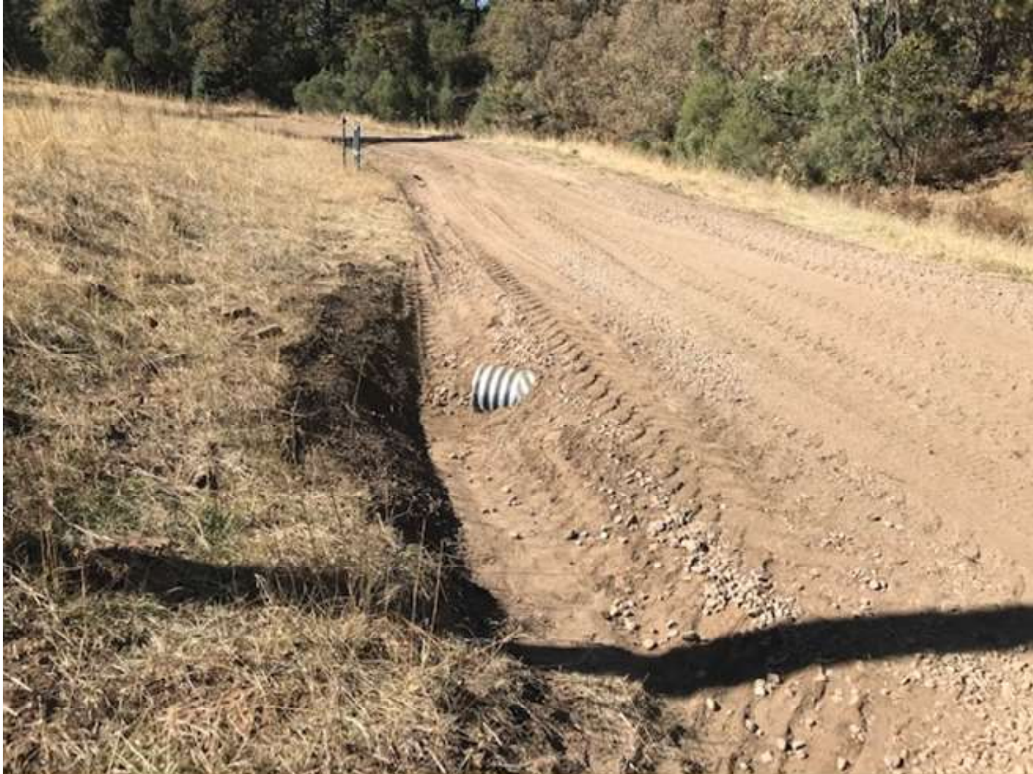
Photo 2: A new culvert was installed where there was some fill slope on the outlet side, to allow enough drop for the culvert to flow stormwater.
