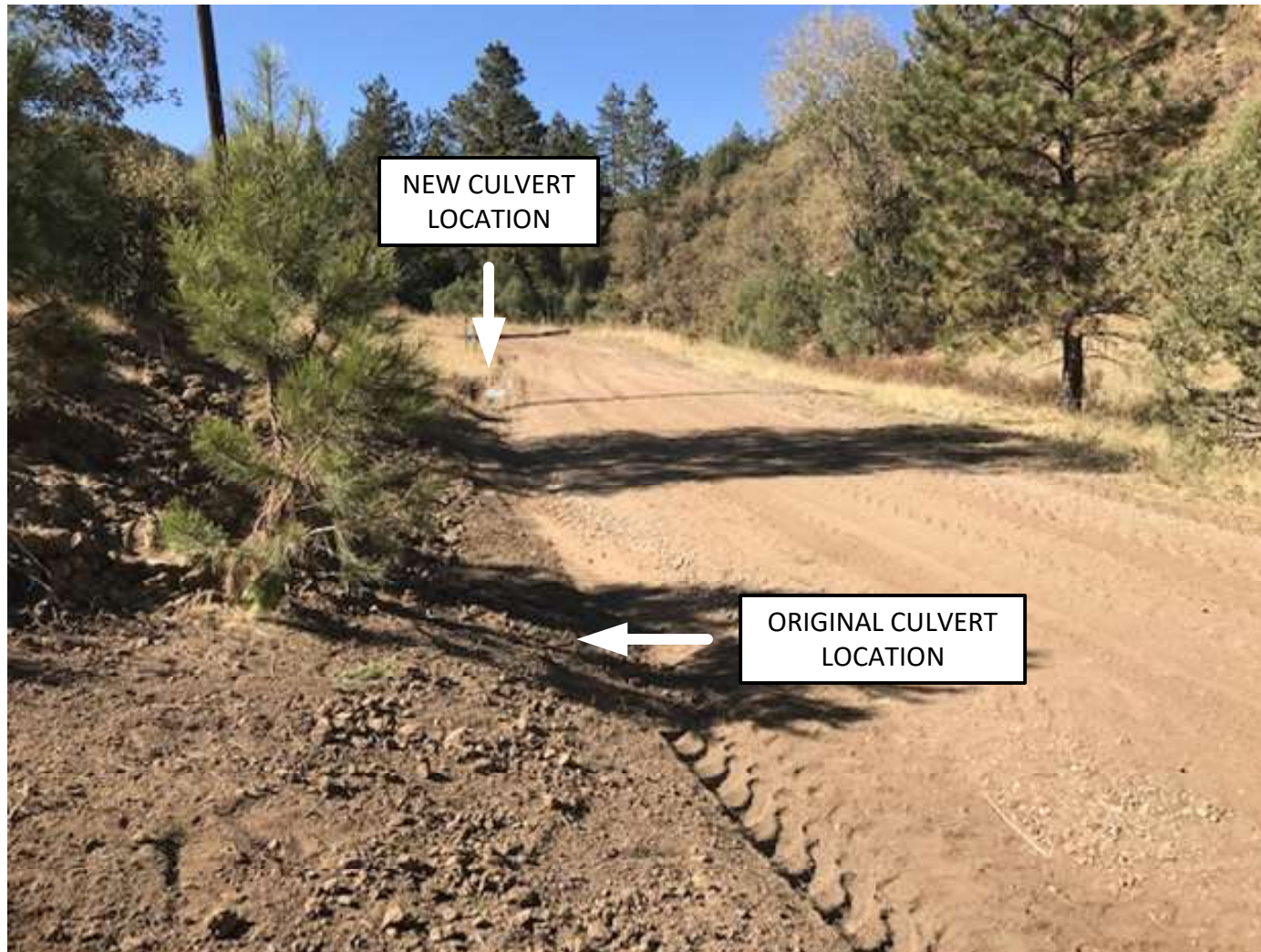
Photo 1: There was no erosion found up gradient of the culvert inlet. This culvert outlet did not have enough drop for the culvert to flow. The culvert outlet had too much vegetation in front of it to flow stormwater out of the culvert. This culvert was removed and a new culvert was installed further up the road.
