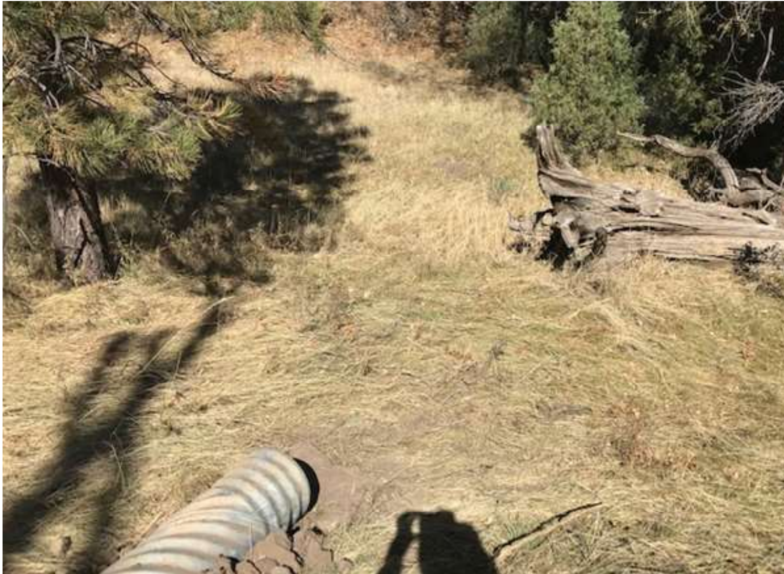
Photo 3: There was enough fill slope for the culvert outlet to be above grade on the outlet side.
