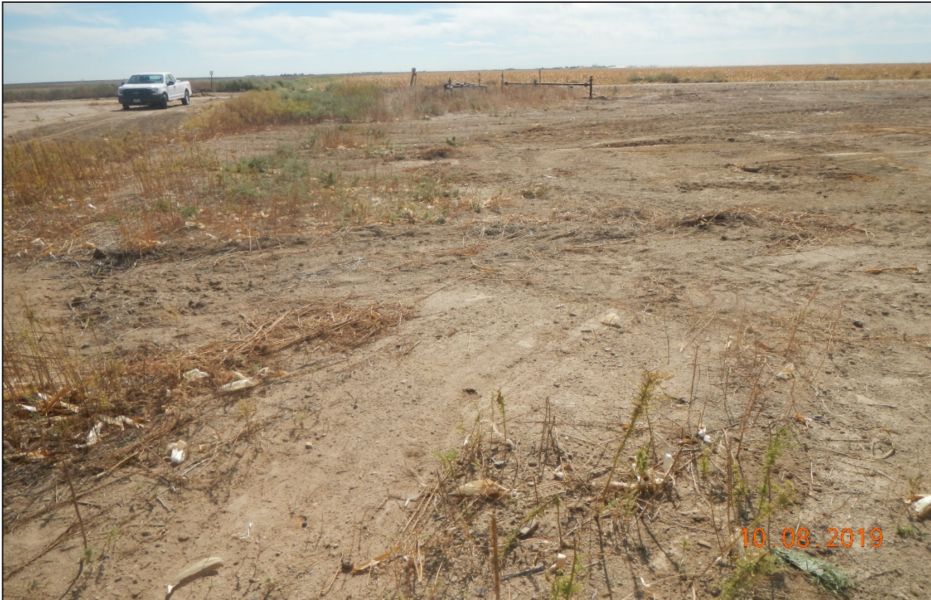
Photo 5. Facing south at the east side of the location. The pipe risers and cement pads have been removed from this area. There was some debris that remains.
