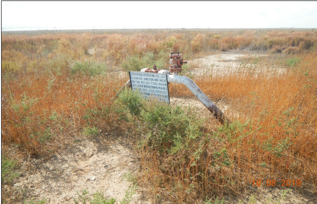
Photo 7. There is a clean out junction north of the pipeline shown in the previous photo that was associated with the compressor station. The sign is from the former operator and is outdated. The cleanout junction needs to be removed.
