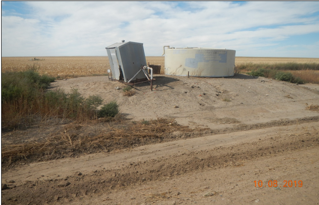
Photo 1. Facing west toward the PW tank and meter shed located adjacent to CR-49 and 575' east of the well. No operator sign installed at the battery site. Corrective actions of the previous inspection were not performed.
