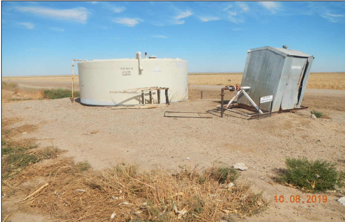
Photo 2. Corrective actions of the previous inspection were not performed. There is no berm around the 200 bbl tank. There is unused equipment at the location.
