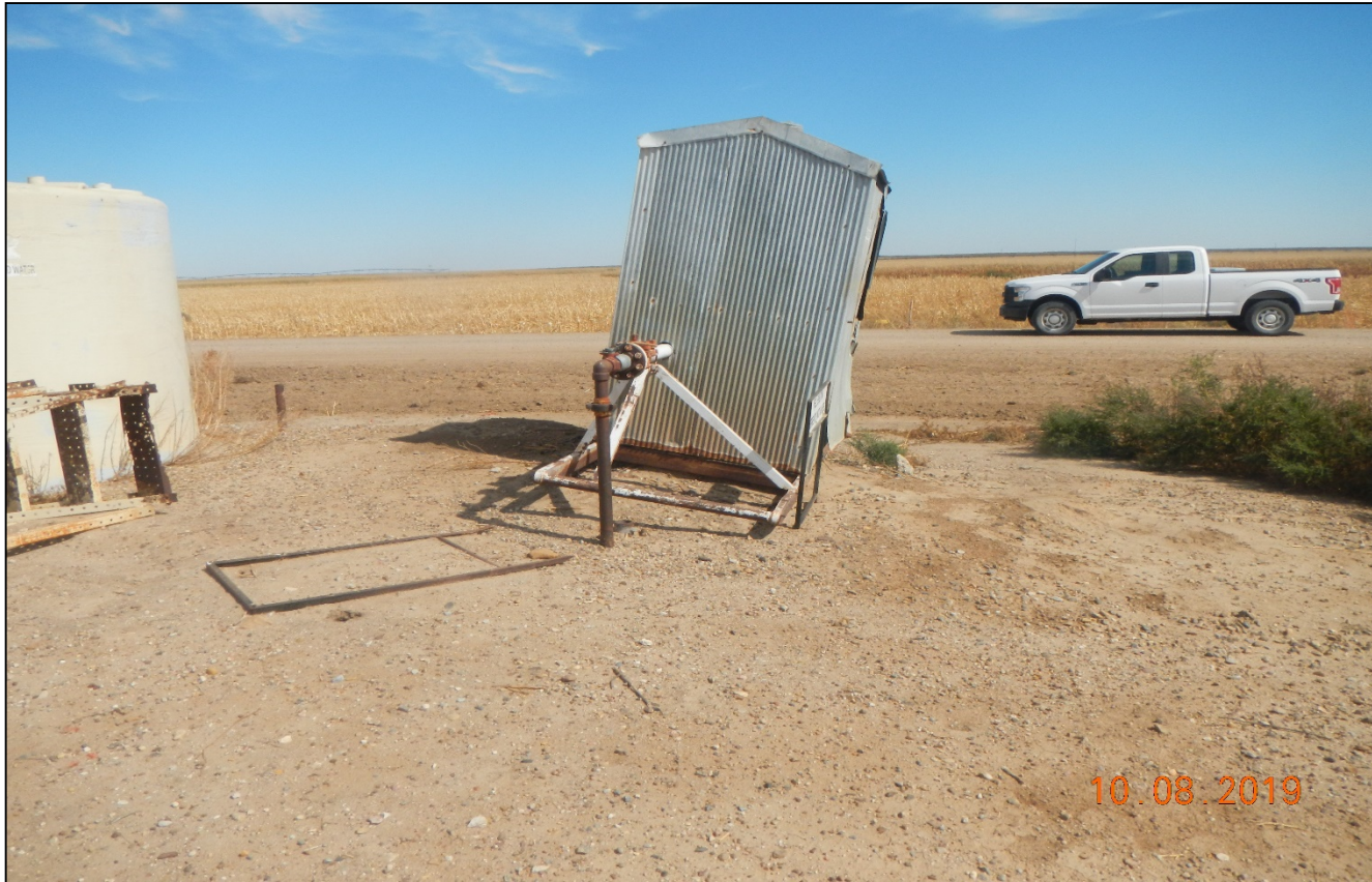
Photo 3. The meter shed does not appear to be stable and is leaning over which is a safety concern. Corrective actions of the previous inspection were not performed.
