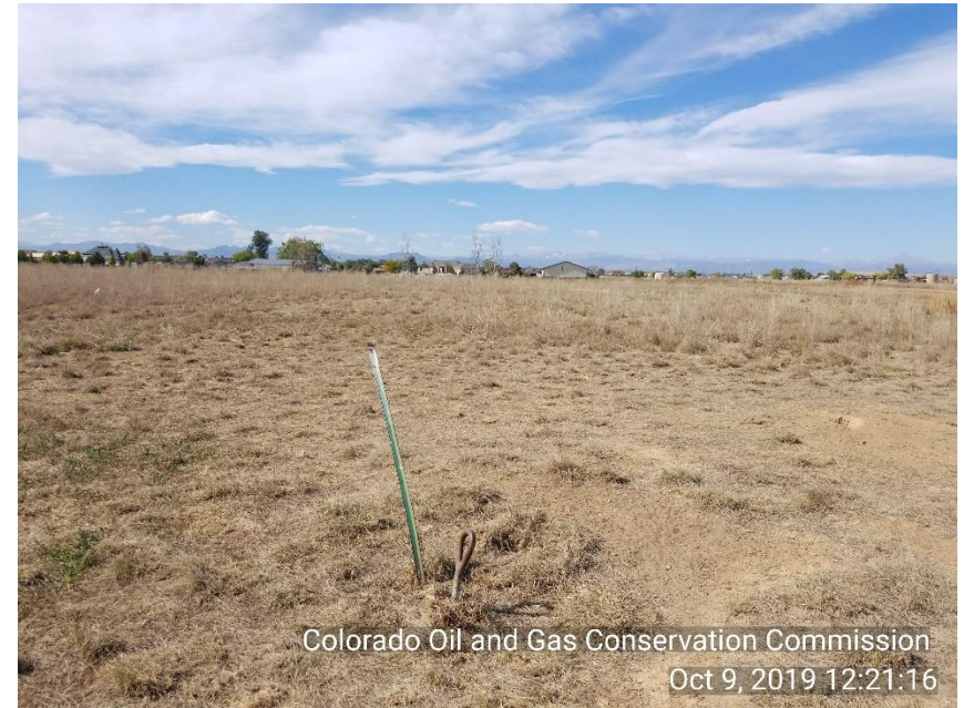
Photo 4 Guy line anchors not properly marked.
