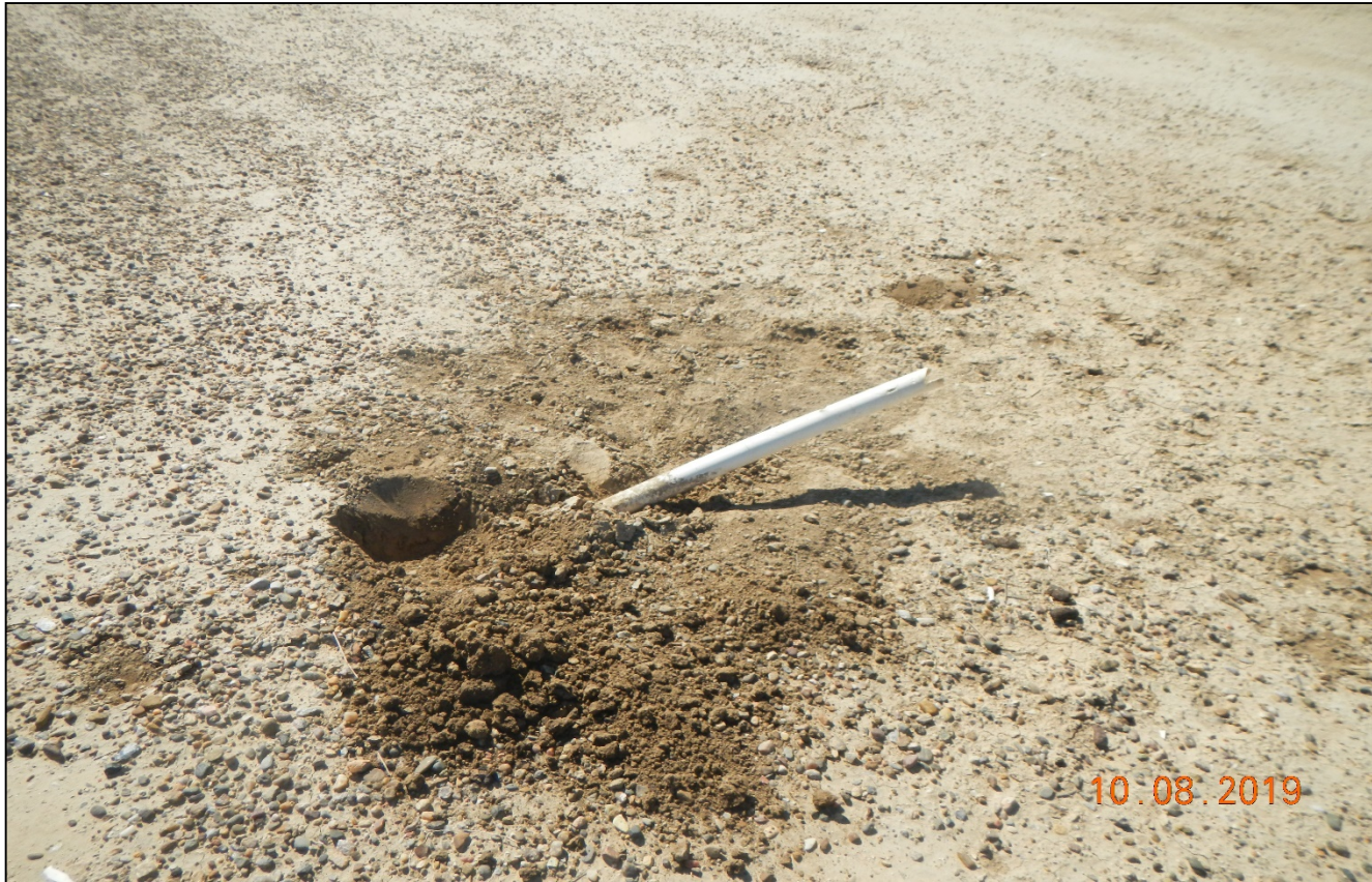
Photo 5. Plastic pipe remains at center of the location. Dug around the pipe but it is buried deep into the ground. Will need to be cut and capped 3 ft. below grade.
