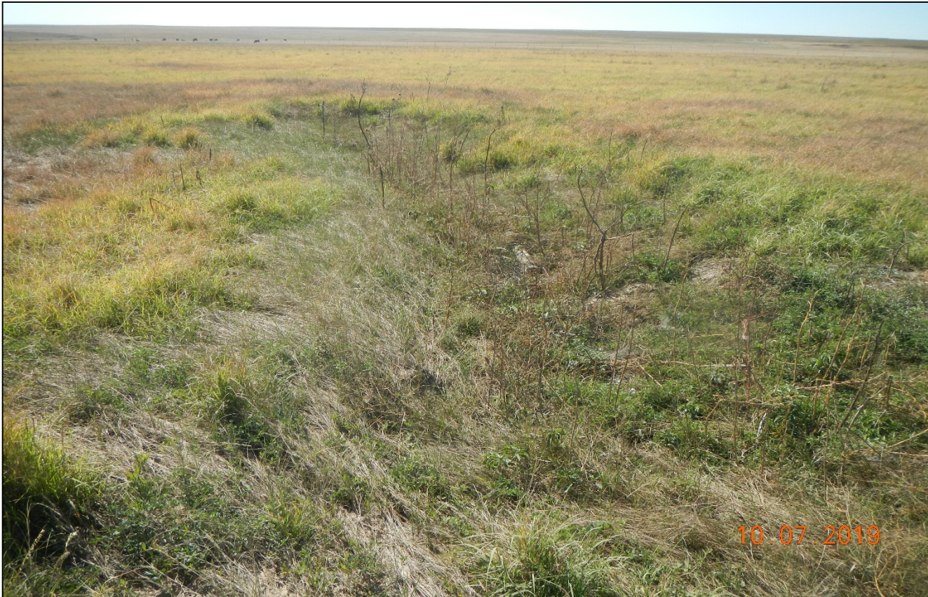
Photo 9. There is an area of subsidence at the west side of the location which is approximately 80 ft. long x 10 ft. wide x 2ft. deep.
