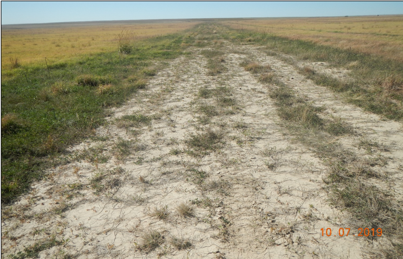
Photo 2. Facing west along the former access road. There are areas along the road where vegetation is not established and soils appear to be compacted.
