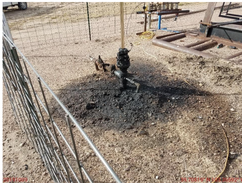
Photo 2: Photo taken from the well, facing south. Photo shows stained soils have not been removed from wellhead. Area of contamination also appears to have expanded since previous inspection dated 5/20/2019.
