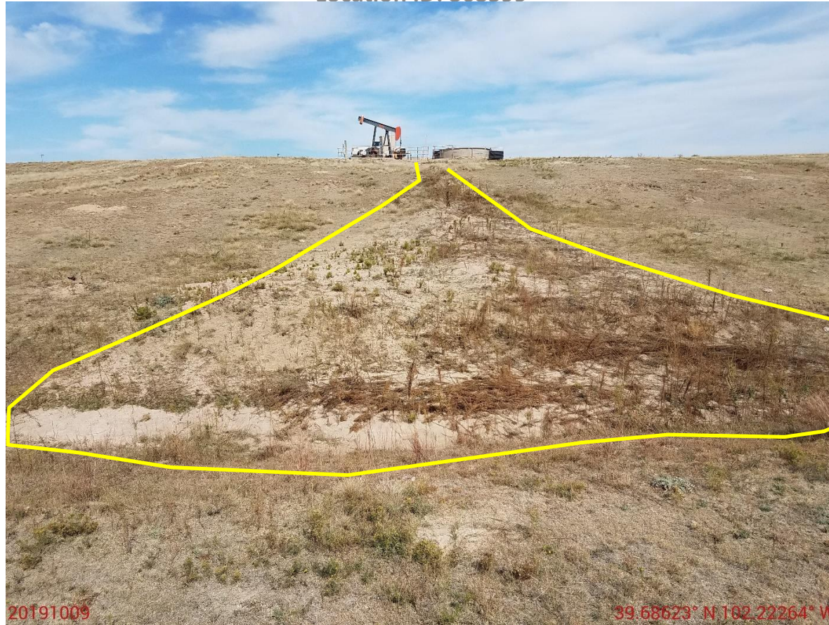
Photo 11: Photo taken from an intermittent drainage south of the location, facing north. Photo shows stormwater runoff from the location has caused degradation to the adjacent lands, as well as sediment deposition in an intermittent drainage/stream. Photo also shows that operator has not conducted reclamation activities to repair the degradation, or installed stormwater and erosion control BMPs.
