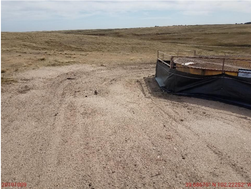
Photo 1: Photo taken from the north end of the location, facing southeast. Photos 1-3 provide an overview of the location from southeast, south to southwest. Photo shows erosion on the pad has been repaired. However, site remains unstabilized and soils loose; location remains at risk to erosion degradation. Photos also show no erosion control BMPs have been installed per CAS
