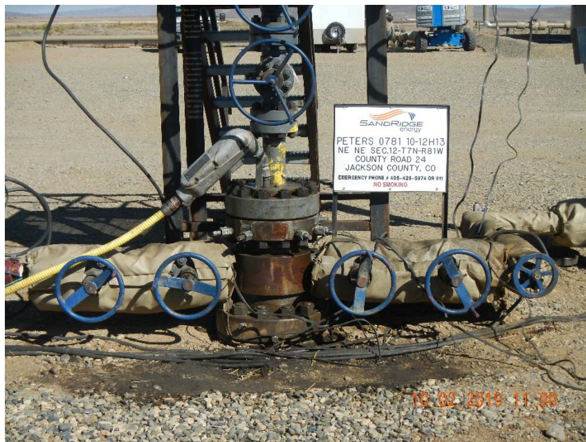
Photo 3. Stained soil at wellhead.
