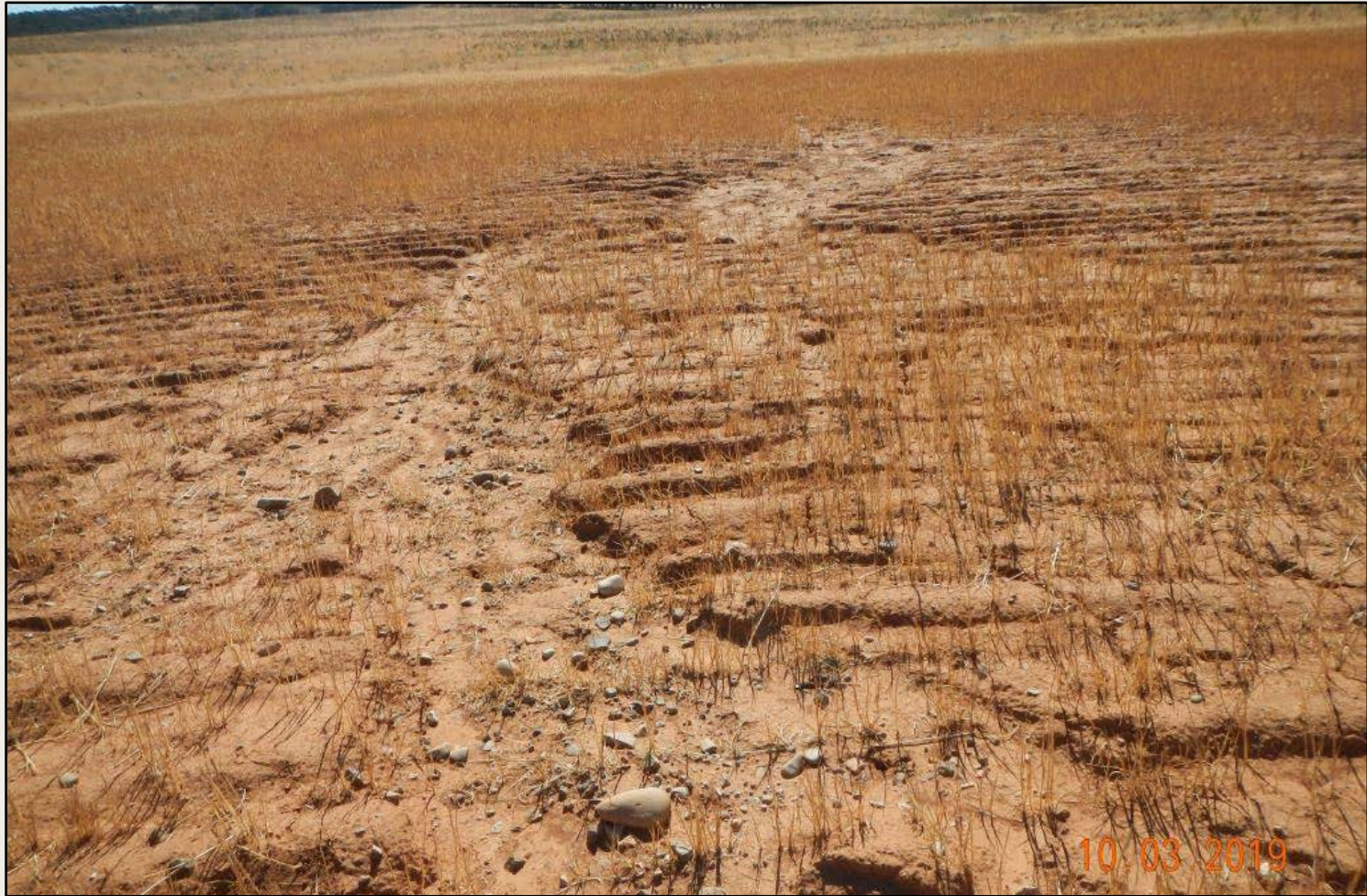
Photo 3. View of erosional channeling (approx. 2 feet wide and 4 inches deep) in eastern and southeastern interim reclamation area, from concentrated stormwater flows exiting the eastern edge of the well pad.
