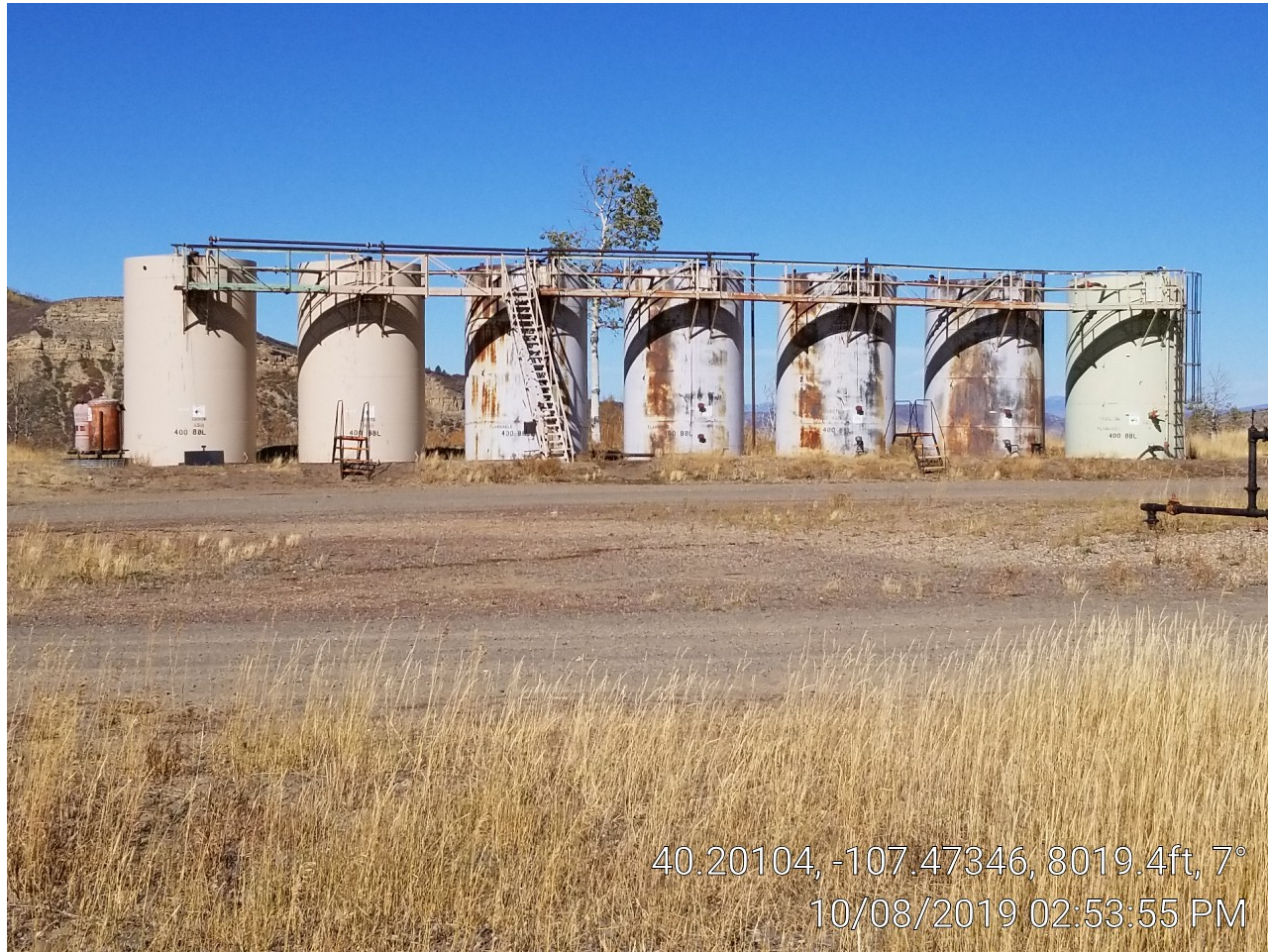
Photo 2. Tank battery.
