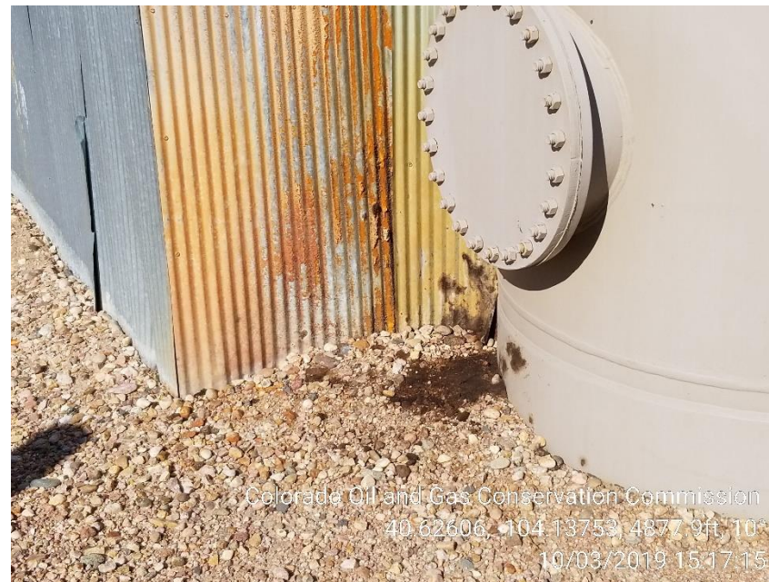
Photo 6 – Stained Soil at Heater Treater
