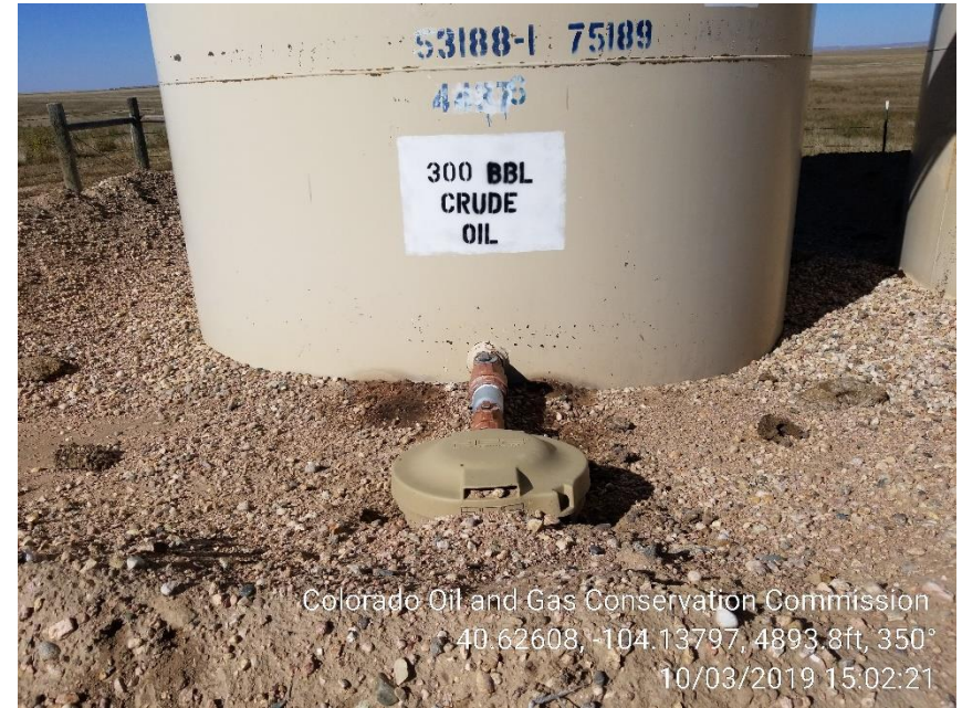
Photo 8 – Stained Soil at West loadline bucket
