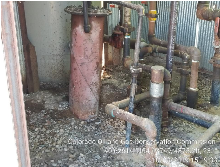
Photo 7 – Stained Soil inside Heater Treater shed
