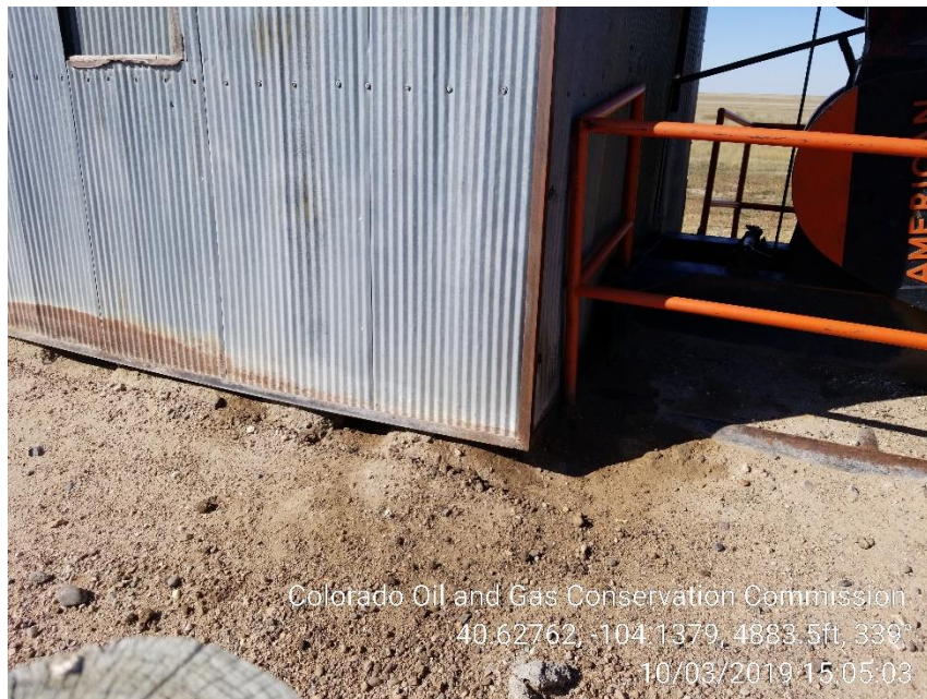
Photo 5 – Stained Soil at Pumping Unit
