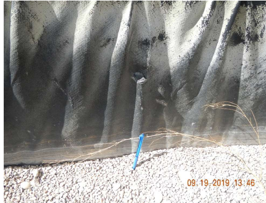
Photo #4 – View of the hole in the lower tank battery liner.
