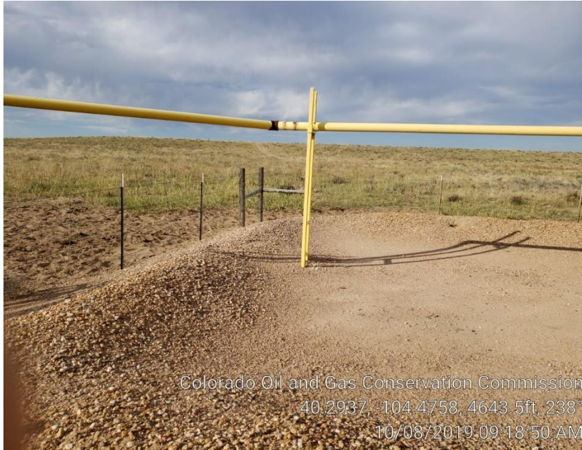
Photo#2 Berm wall weathered
