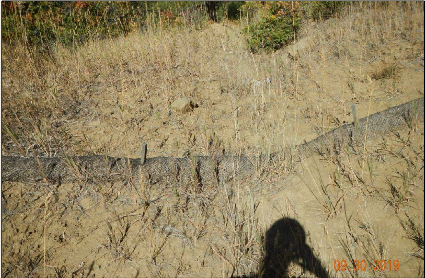
Photo 4. View of another straw wattle that is full of sediment and needs maintenance/repair.
