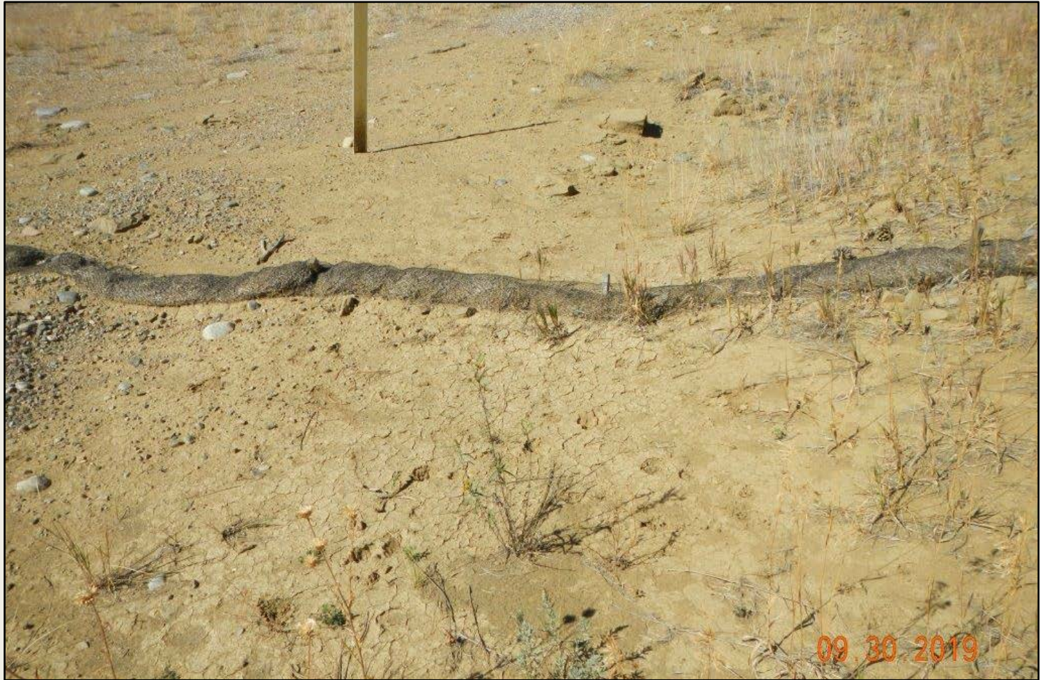
Photo 3. View of straw wattle on the northern edge of the working area, full of sediment and no longer functional.
