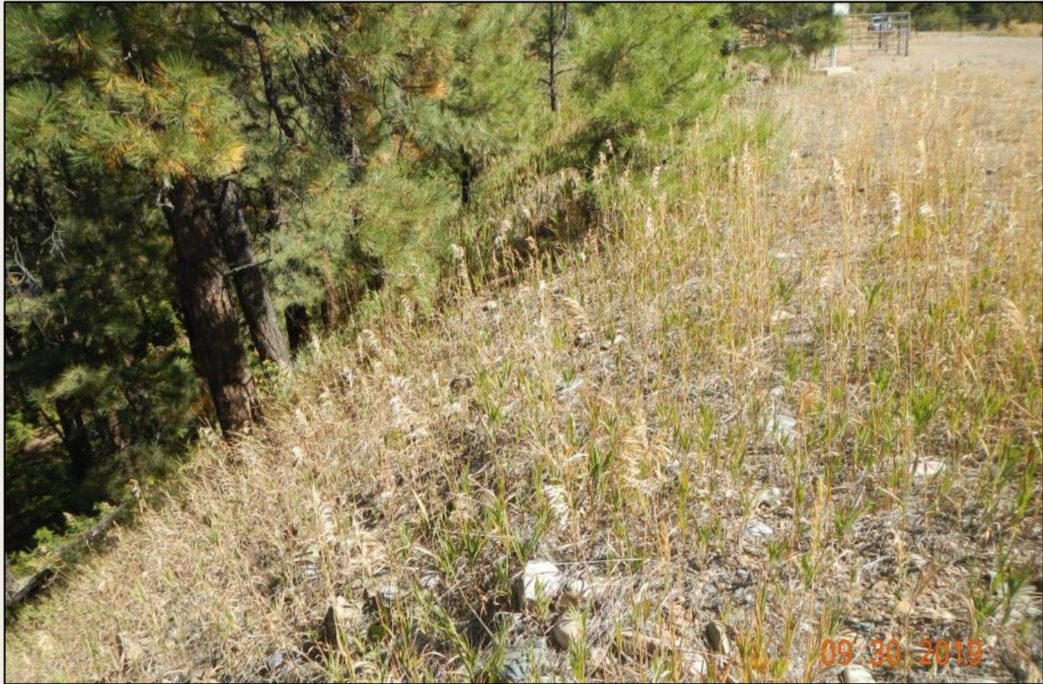
Photo 2. View of the northern portion of the project area from the western edge facing northeastward. Fill slope appears stabilized with grasses such as smooth brome and young ponderosa pine and gambel oak trees.
