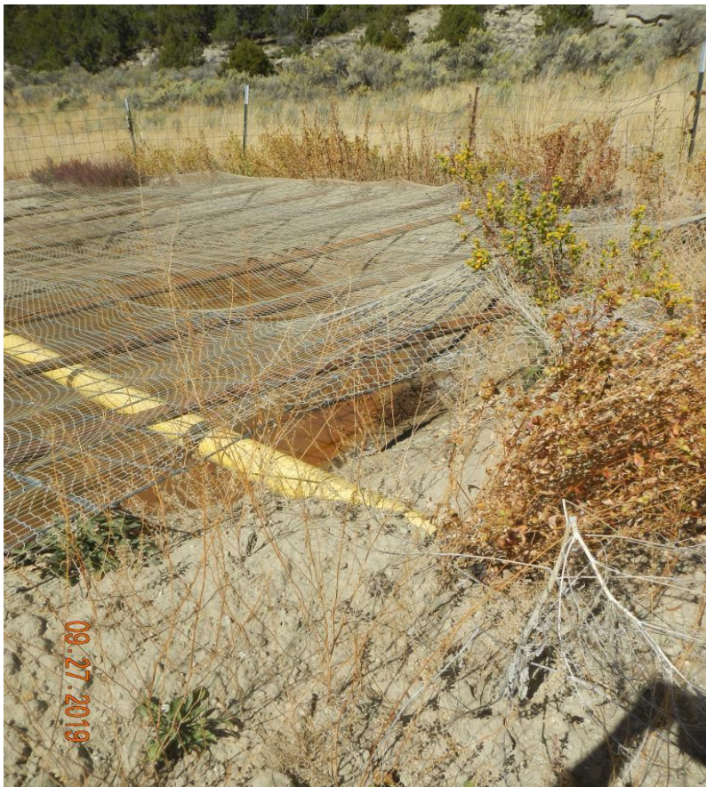
Photo#3: Area of damaged, gaped netting.
