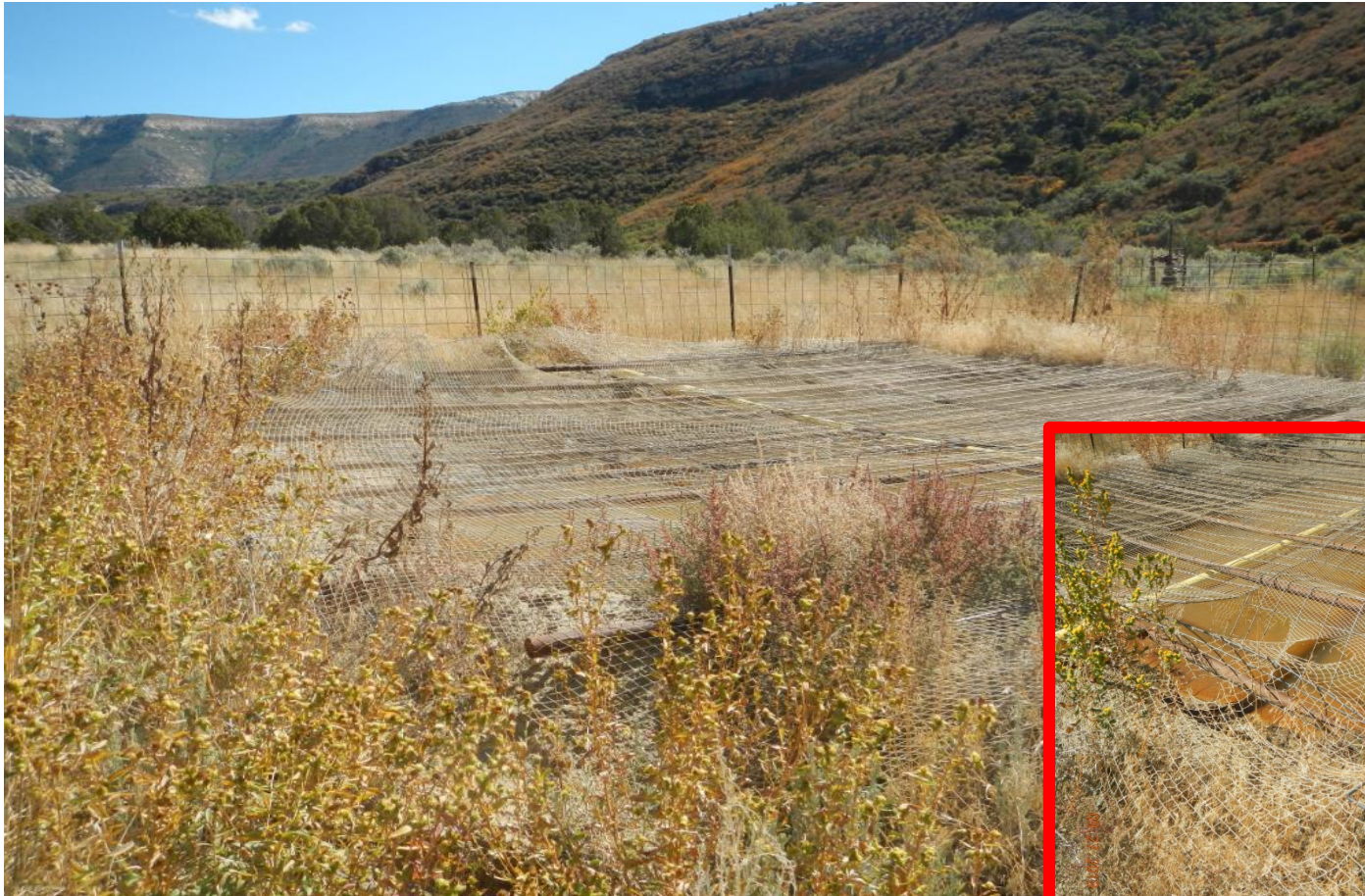
Photo#2: View over Blowdown Pit. Insert showing one area of damaged netting
