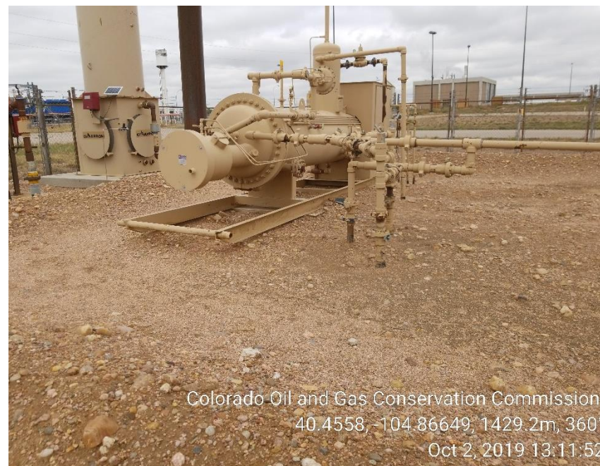
Photo 8: Separator not anchored
