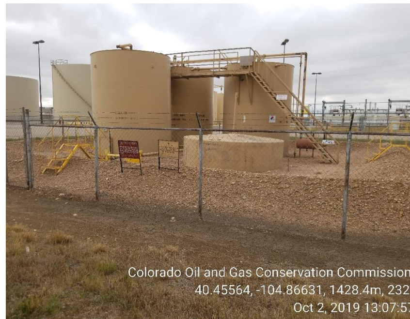
Photo 6: Tank Battery; Inadequate berms, tanks not anchored
