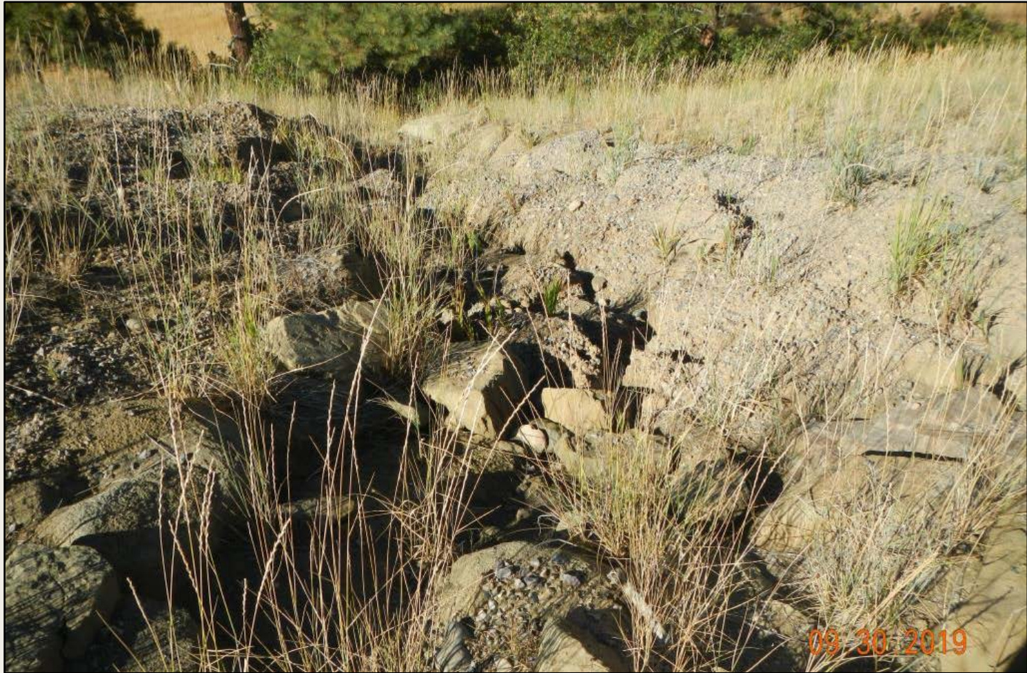
Photo 3. View of erosion occurring around rock BMP within the western project area.
