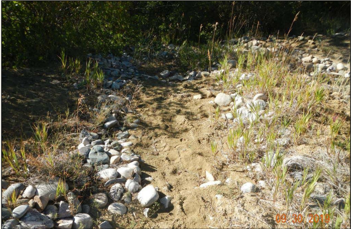
Photo 2. View of sediment accumulation within cobble lined silt trap, needing maintenance.
