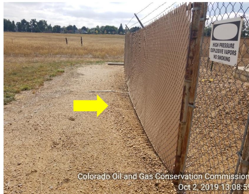
Photo 4 Can see where fence around TNK BTRY is rubbing on the ground from what appears to be the wind
