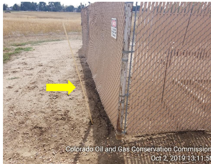
Photo 8 Can see where fence around sep/meter house is rubbing on ground from what appears to be the wind.
