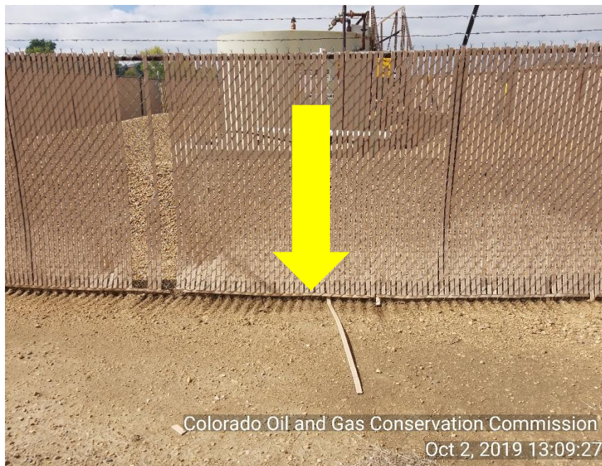
Photo 5 Can see where fence around TNK BTRY is rubbing on the ground from what appears to be the wind
