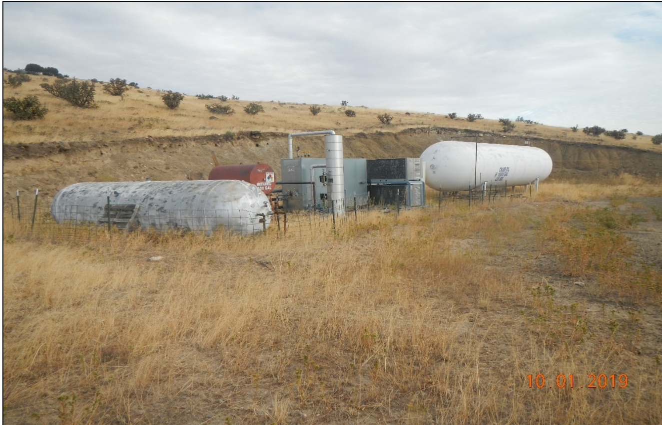
Photo 4. Facing towards the storage tanks. The berm appears to be inadequate and there is dry vegetation around the tanks which is a fire hazard.
