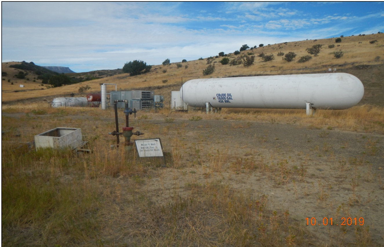
Photo 5. The sign at the well head does not display an emergency contact number, operator number, and public road description.
