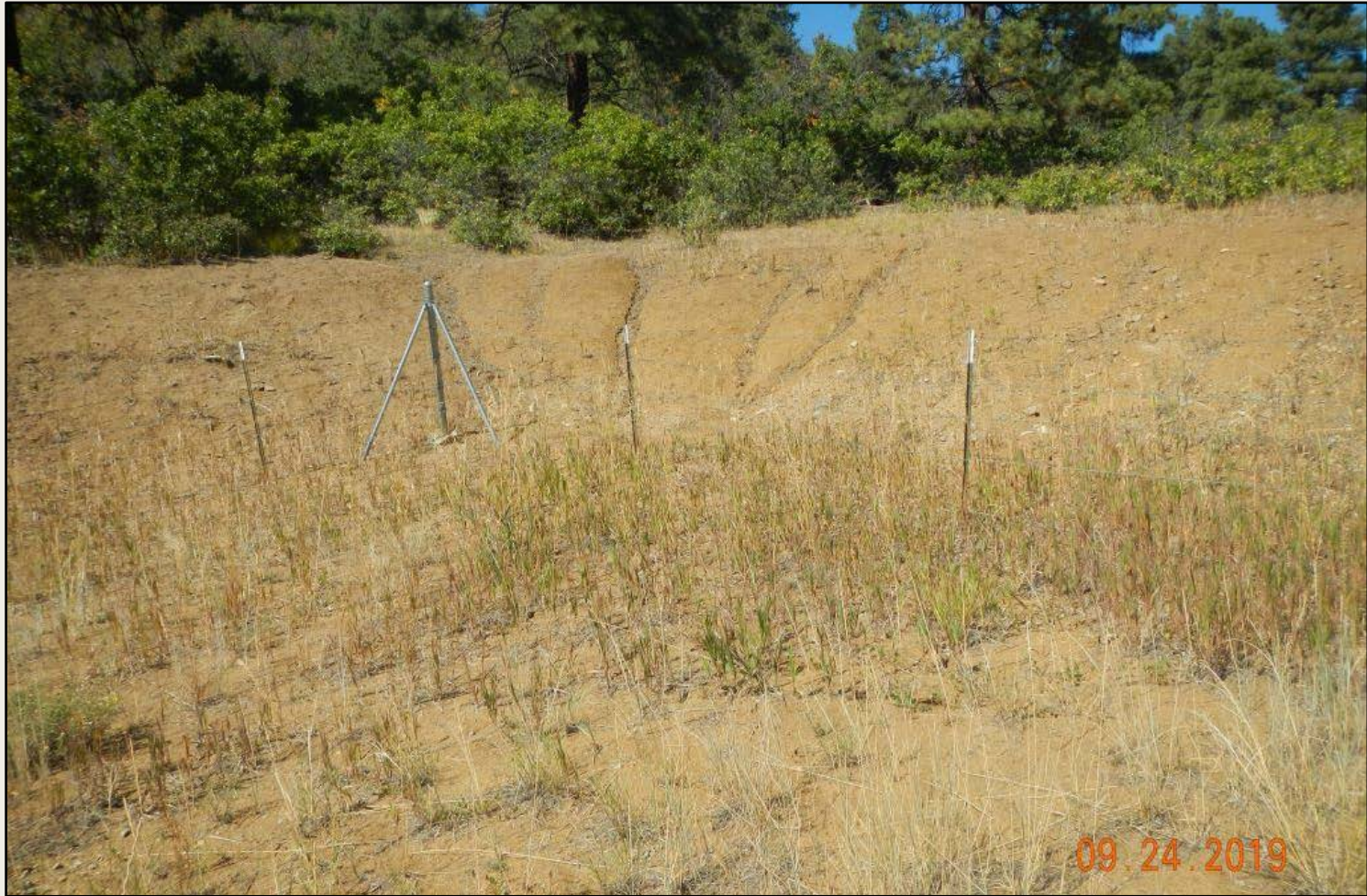
Photo 3. View of erosion occurring on the northwestern project area. Significant sediment deposition observed down-slope. Bare soils on slope are not stabilized.
