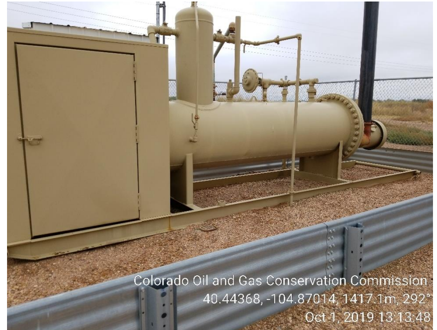
Photo 6: Separator not anchored
