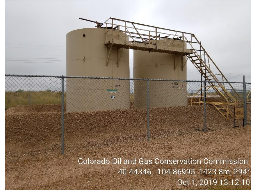
Photo 4: Tank Battery; TANKS NOT ANCHORED, EARTH BERM
