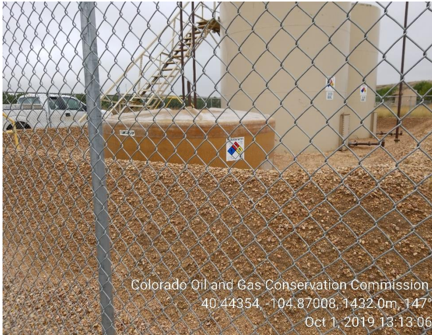
Photo 5: NO BBLs LABELED ON PRODUCED WATER, EARTH BERM, TANK NOT ANCHORED
