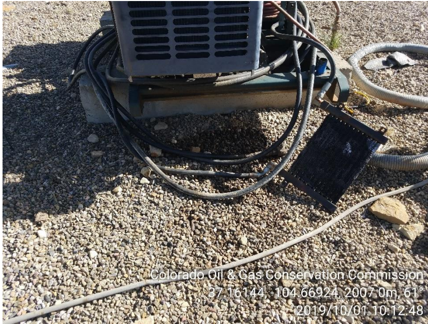
PHOTO 3: OILY STAINED SOIL NEAR ENGINE SKID. Properly treat or dispose of oily waste in accordance with 907.e. CA DATE 11-1-19
