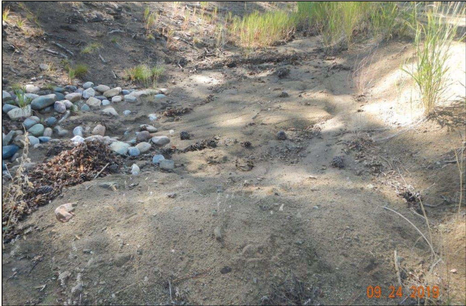
Photo 2. View of sediment catchment within the eastern project area needing maintenance. Additional BMPs to prevent sediment run-on are recommended.
