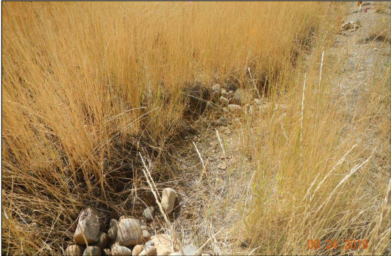
Photo 2. View of cobble in ditch along access road. Cobble placed in this manner is not a BMP installed in accordance with good engineering practices. See CDOT erosion control and stormwater quality field guide for examples. This will need to be carefully monitored and if erosion continues here additional BMPs will need to be installed using good engineering practices.
