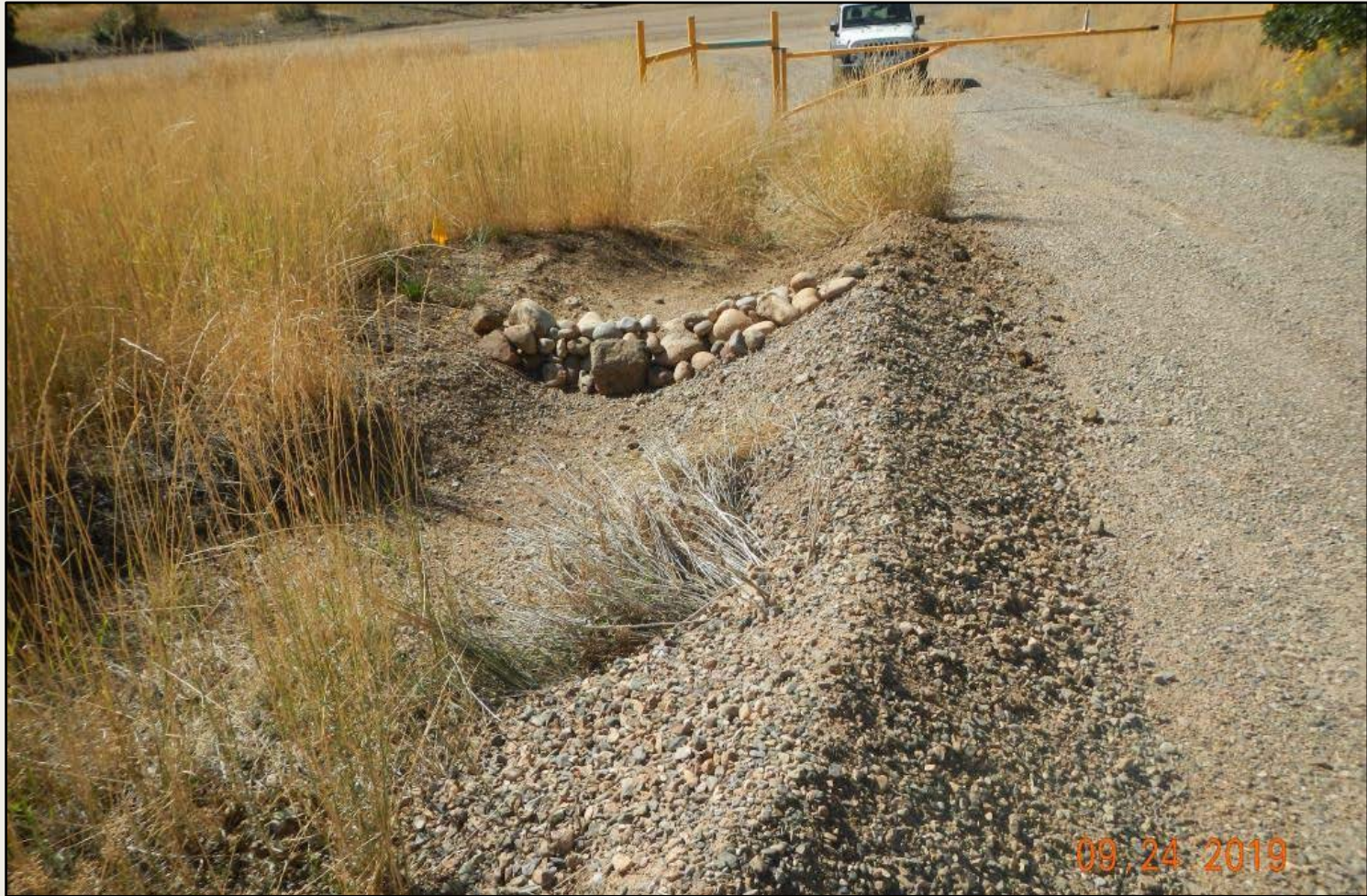
Photo 1. View of repaired ditch and berm along the access road entrance.
