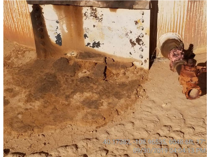
Photo 3. Stained soil at tank.
