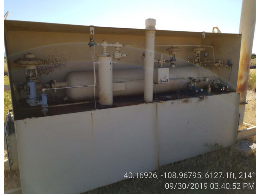
Photo 3. Horizontal separator.
