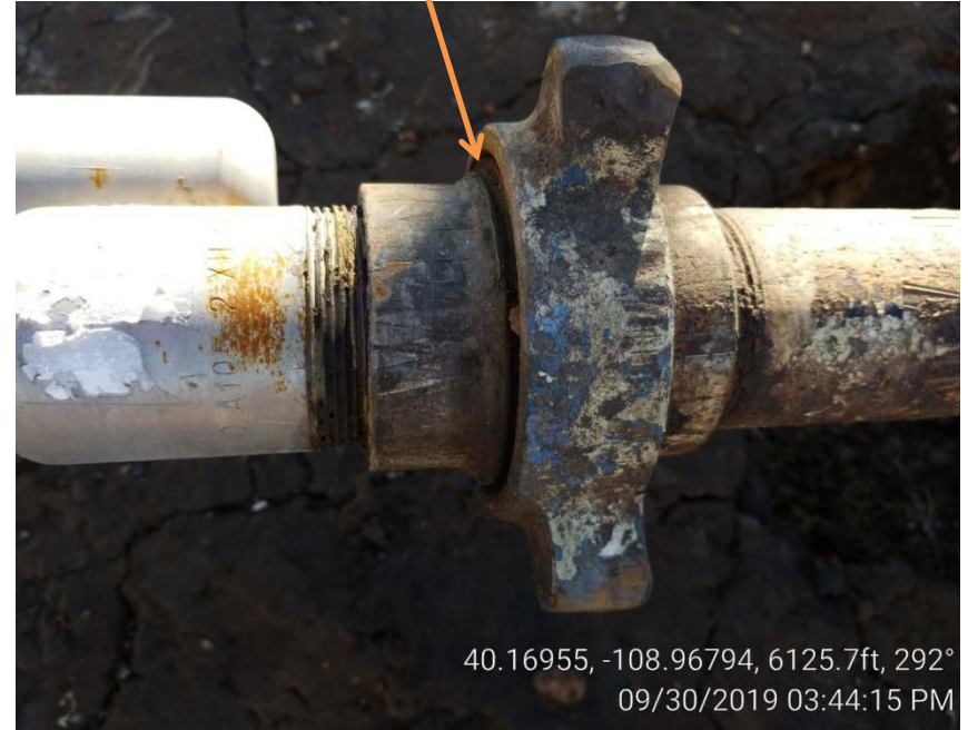
Photo 11. Gas leak.
