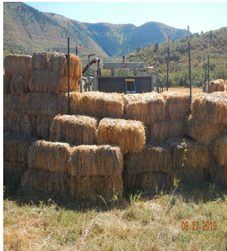
Photo#4: View outside of sound wall; top layer of bales not in place.
