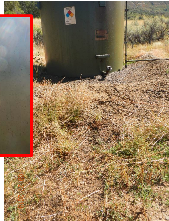
Photo#18: Staining observed outside of tank berm.
