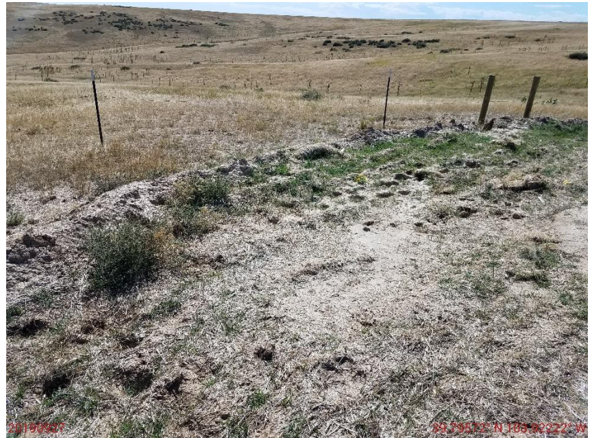
Photo 4: Photo taken from the south end of the location. Photo shows operator has installed a berm. Berm remains loose and unconsolidated material. BMP has not been installed in accordance with good engineering practices.
