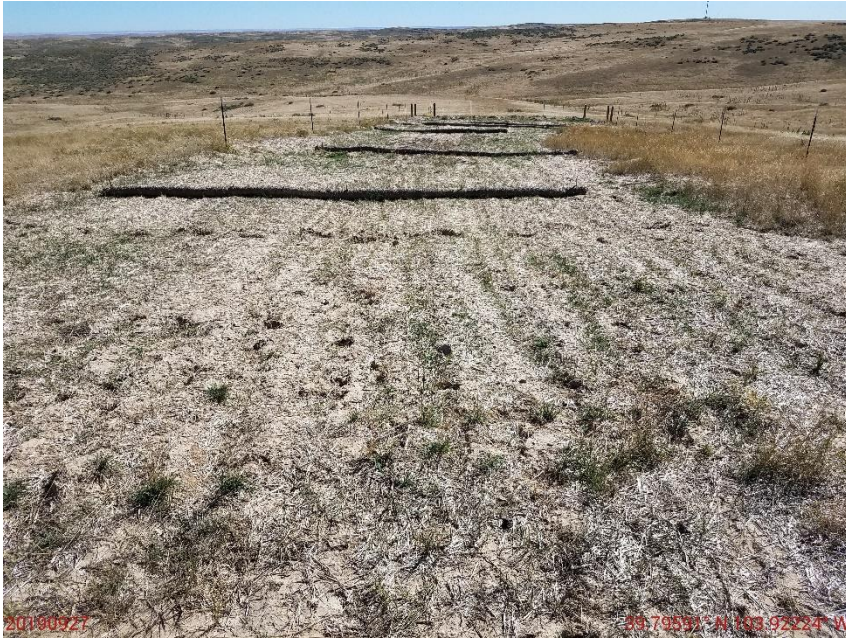
Photo 1: Photo taken from the north end of the location, facing south. Photo shows additional reclamation appears to have been conducted, however, operator has seeded up the slope rather than along the contour. Seeding actives have not been conducted in accordance with good engineering practices and will likely facilitate erosion degradation.
