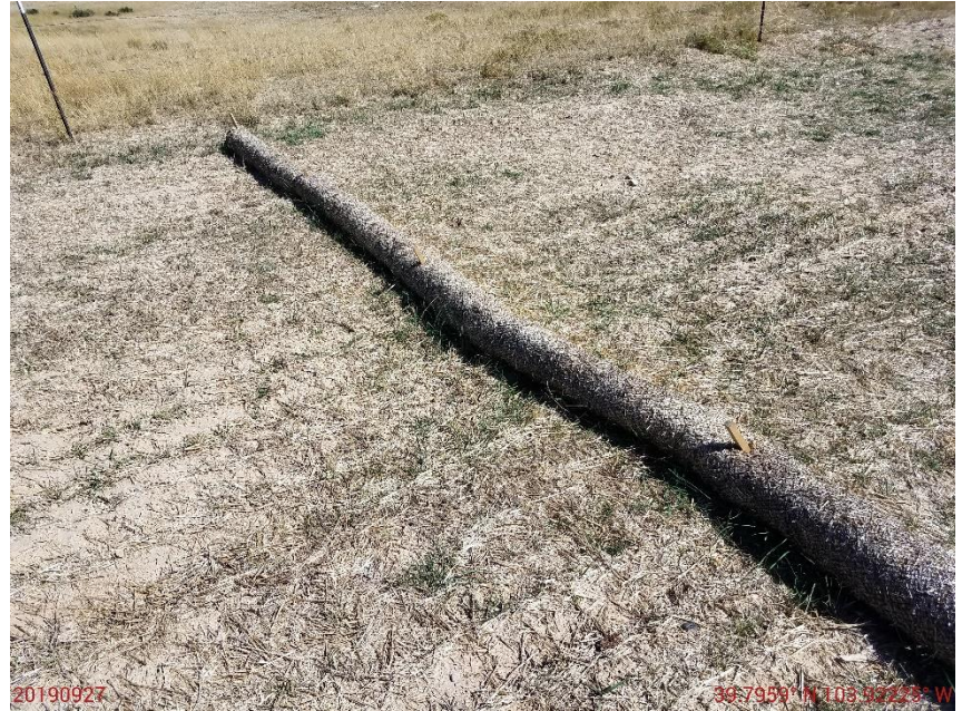
Photo 2: Photo shows wattles on location have not been properly staked/trenched/backfilled in accordance with good engineering practices. BMP is not in proper functioning condition.
