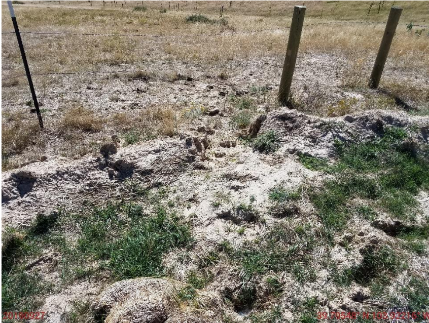
Photo 5: Contined from photo 4. Photo shows area of the berm that has been “blown-out”. BMP is not in proper functioning condition.
