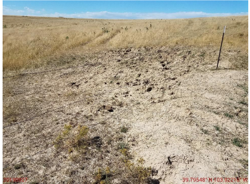
Photo 6: Photo taken from the south end of the location, facing west. Photo shows areas to the west of the location where stormwater runoff from location deposited sediment. It does not appear as though these areas have had additional reclamation activities conducted, or BMPs installed.
