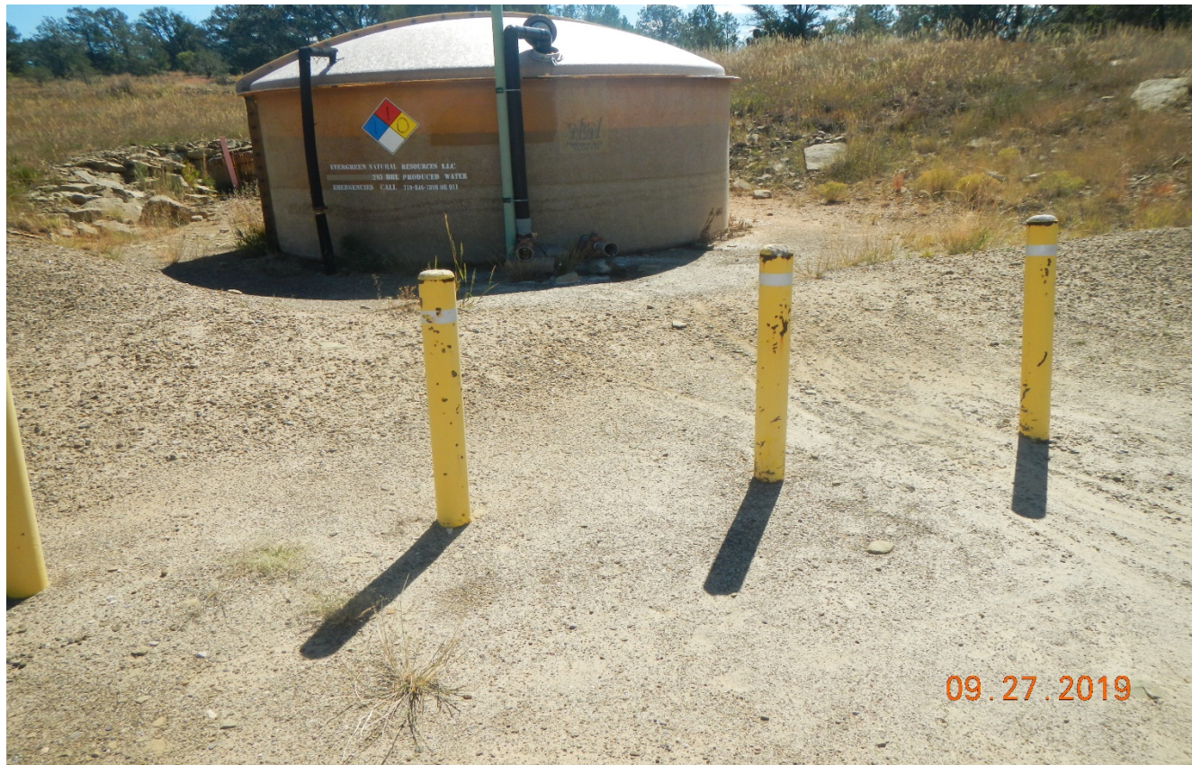
Photo 2. The berm around the tank is worn down and appears to be inadequate to contain spill.
