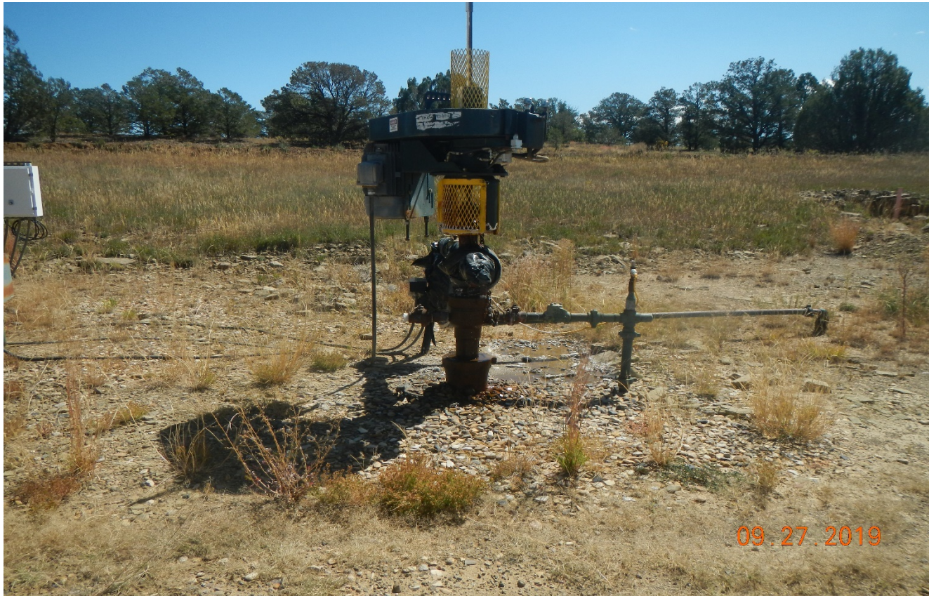
Photo 1. There is a dripping water leak at the wellhead.
