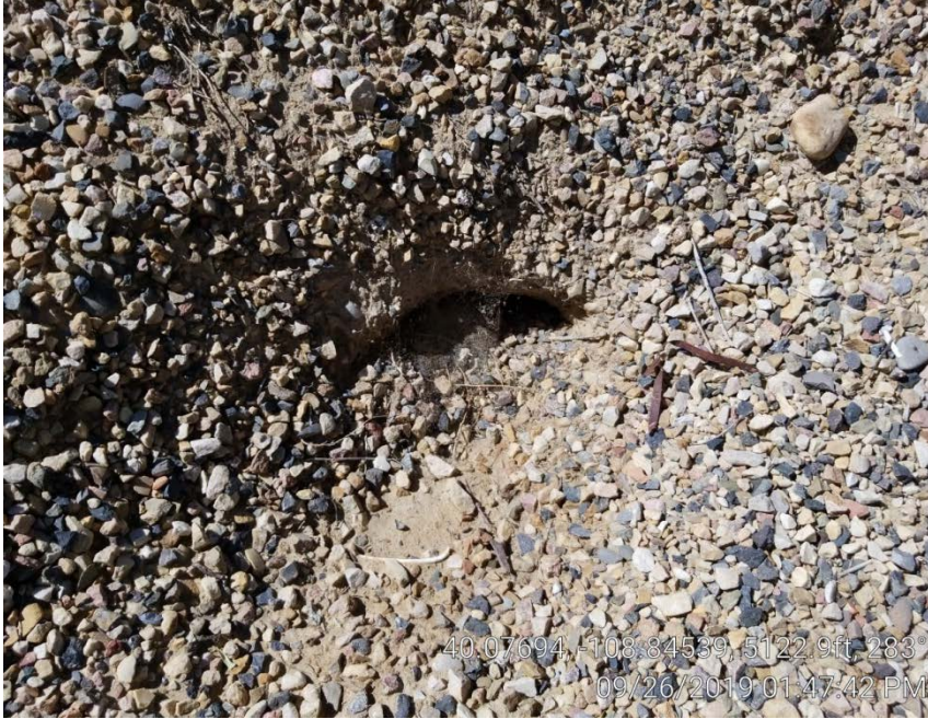
Photo 4. Animal burrow hole inside of west tank berm.
