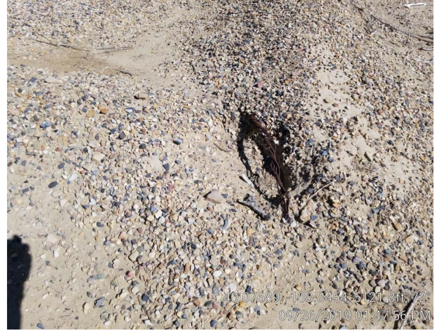
Photo 5. 1' wide low spot in berm SW corner.
