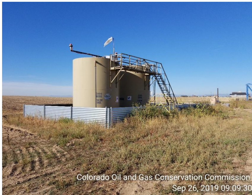
Photo 5 TNK BTRY Weeds in and around containment. No BTRY sign.
