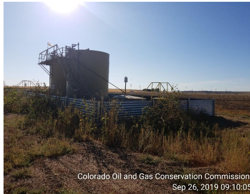
Photo 6 TNK BTRY Weeds in and around containment. No BTRY sign.
