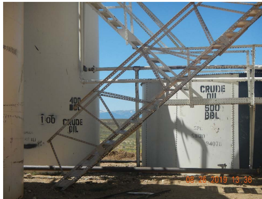
Photo 8. Incomplete tank labels, no NFPA diamond.
