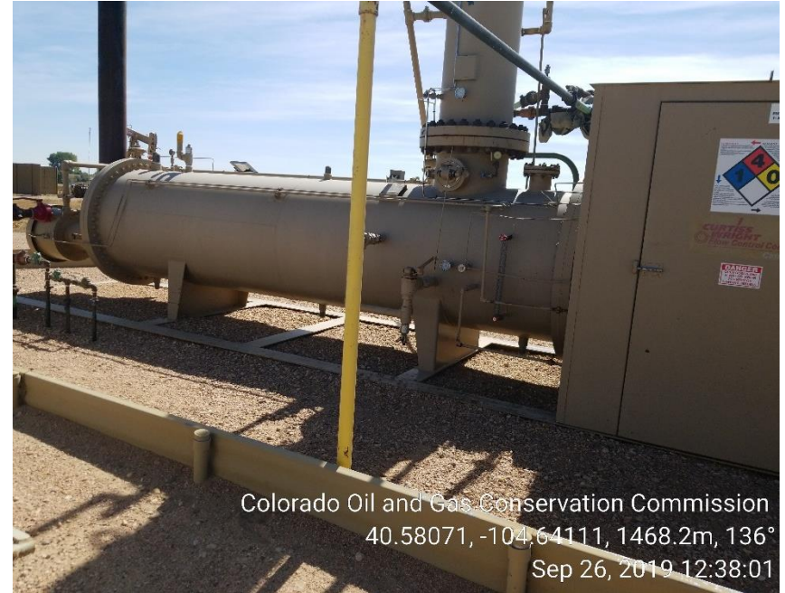
Photo 6: Separator not anchored
