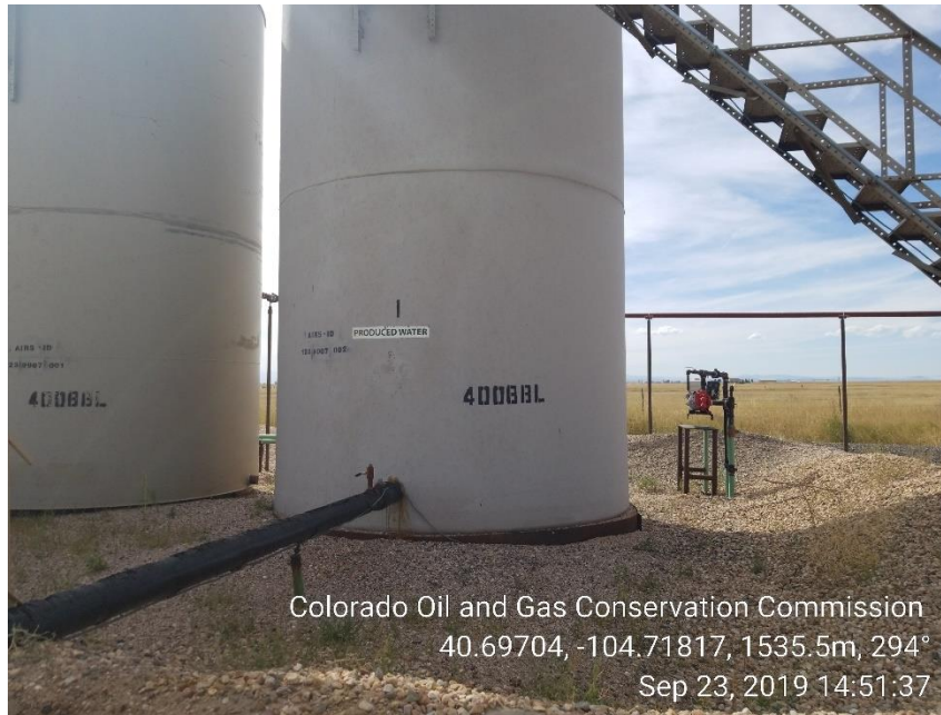
Photo 7: No NFPA Placard on H2O tank
