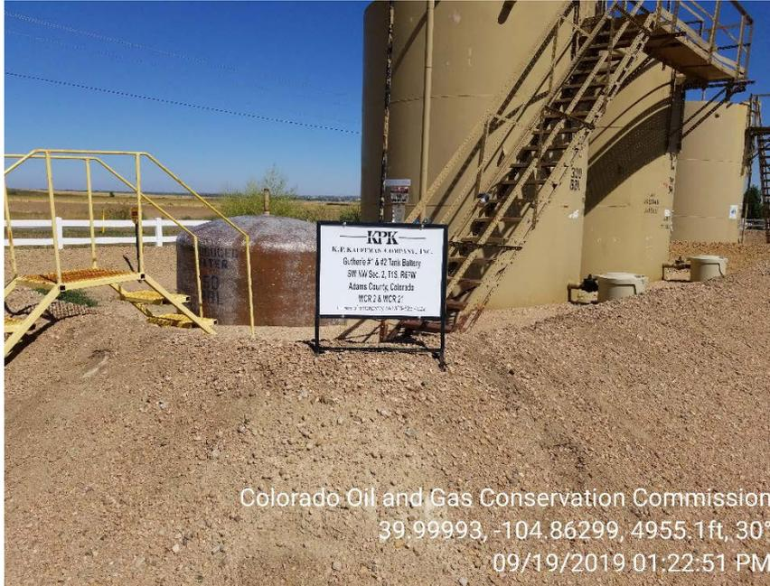
Photo 1 – Tank Battery Sign; fiberglass produced water tank on site
