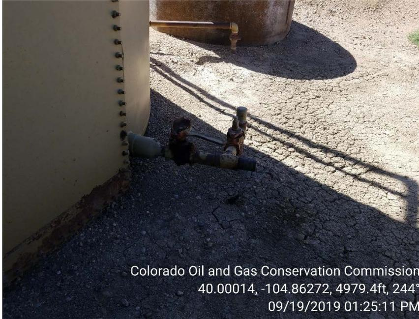
**Photo 5 – Stained soil under crude oil tank valve**
