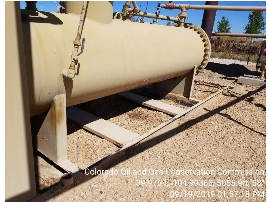
Photo 8 – Stained soil under separator
