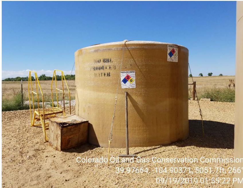
Photo 3 – Location photo; fiberglass produced water tank on site
