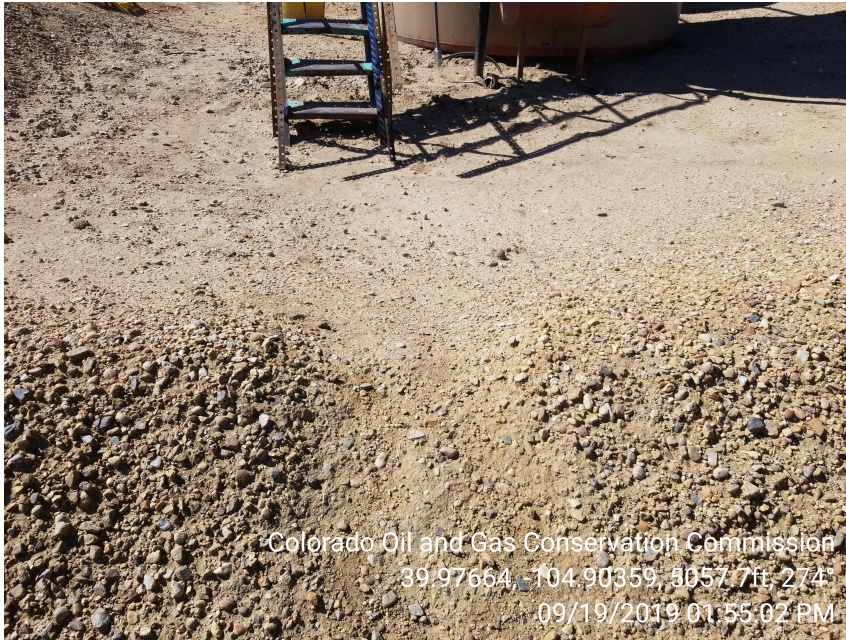
Photo 5 – Berms around tanks in disrepair
