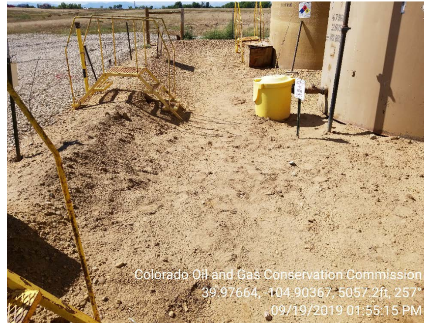
Photo 4 – Berms around tanks need repair
