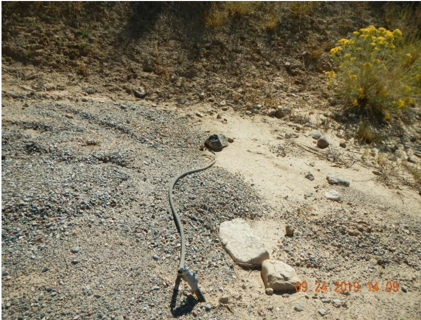
Unused electrical conduit with wiring at base of cut slope between separators and tanks.
