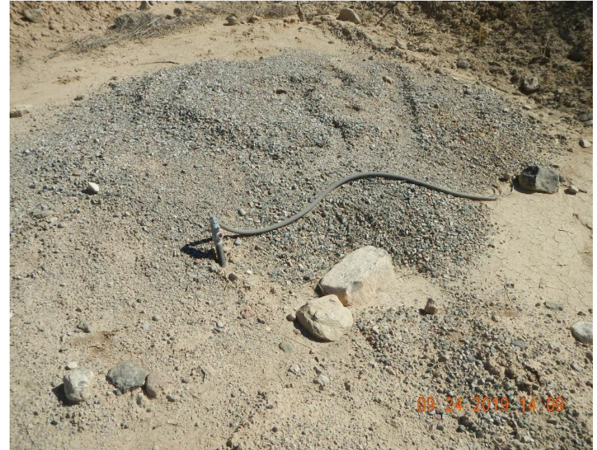
Unused electrical conduit with wiring at base of cut slope between separators and tanks.
