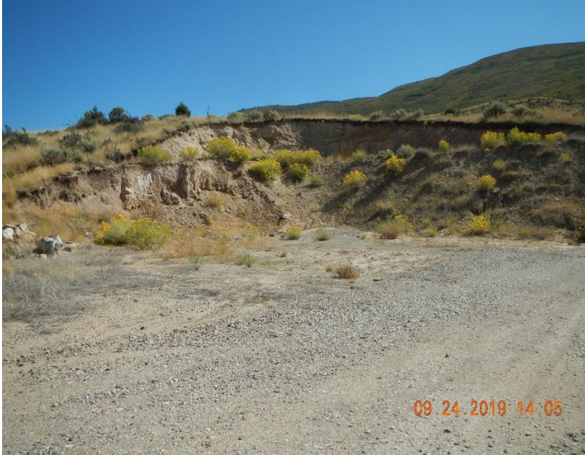
Unstable cut slope between separators and tanks with sediment movement.
