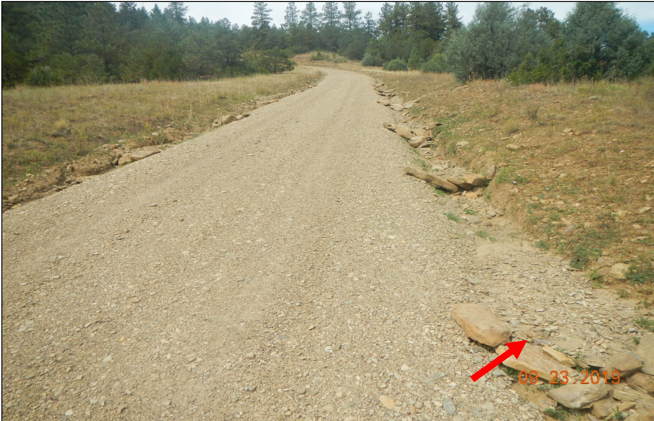
Photo 1. Gravel has been spread along the access road. Rock check dams are installed. Some of which are filled in with sediment and need maintenance.
